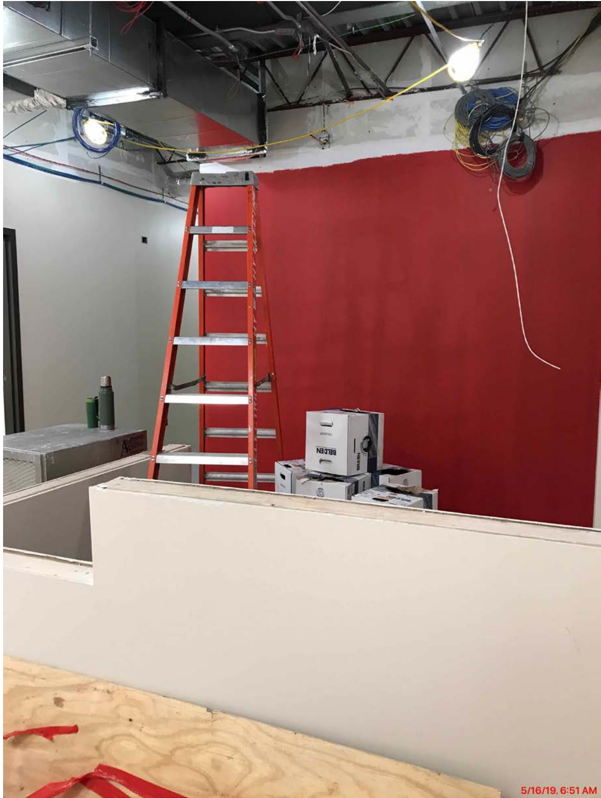
District Office Reception Area Installation and Painting Begins
