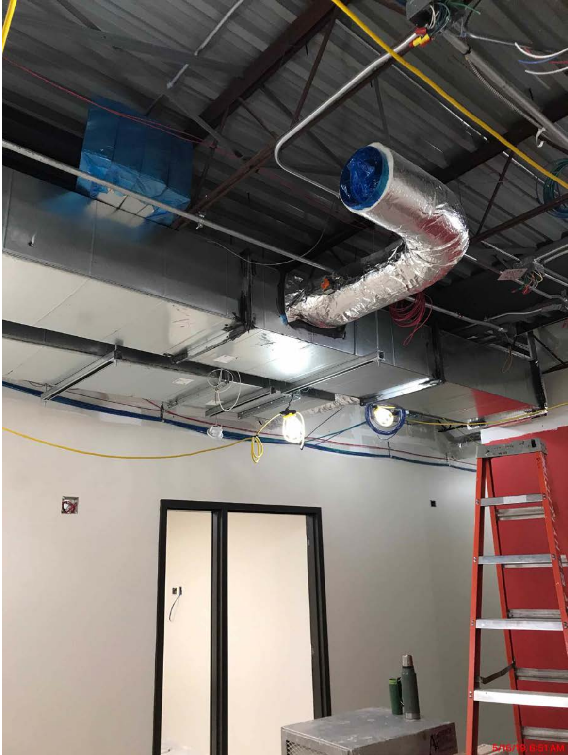
Duct Work Installation at District Office
