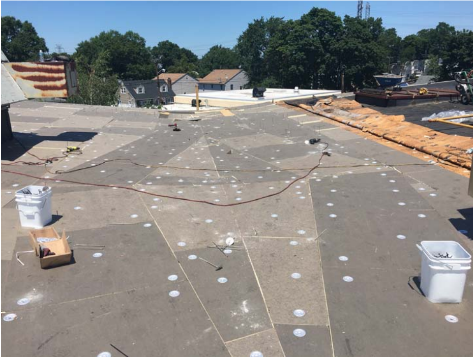
July 2018: Belleville HS –Tapered Insulation being installed at HS Roof C.
