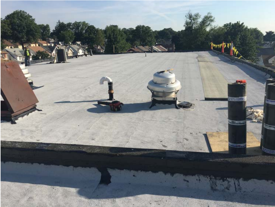
July 2018: Belleville ES #3 – Cap sheet installation substantially completed at Roof A2.
