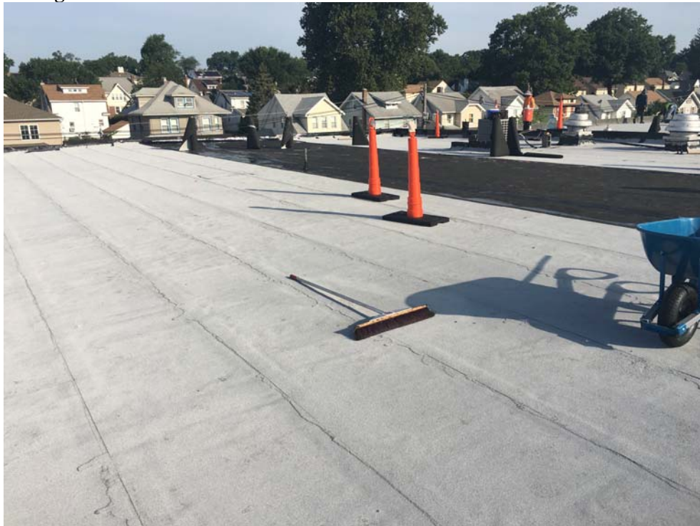
July 2018: Belleville ES #3– Ongoing Cap Sheet Installation at Roof A1.
