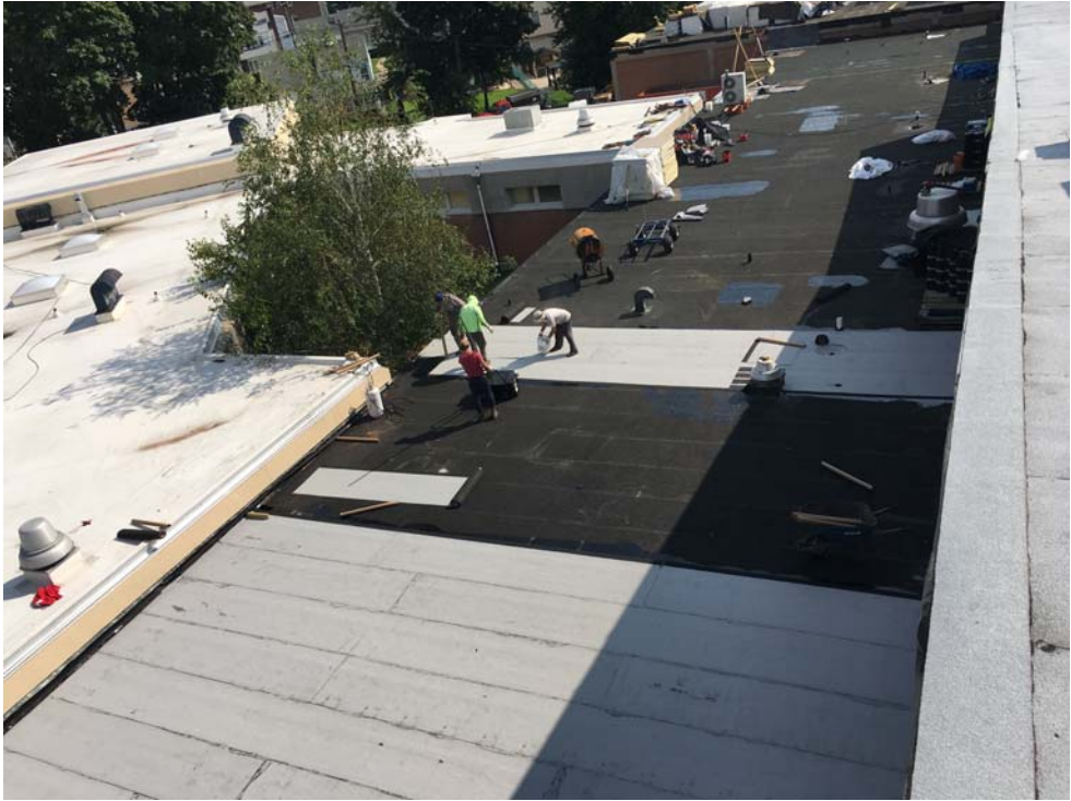
August 2018: Belleville HS – Ongoing Cap Sheet installation at Roof D.
