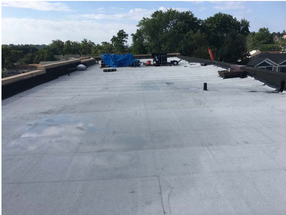
August 2018: Belleville ES #9 – Cap sheet installed on high Roof B.
