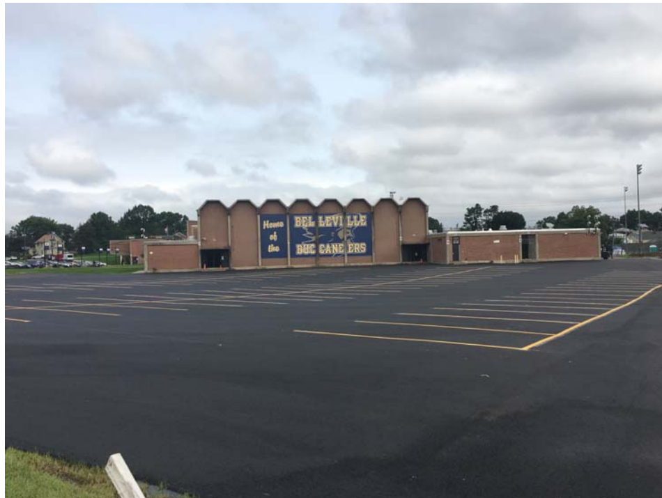
August 2018: Belleville HS – Striping installed at high school parking lot.
