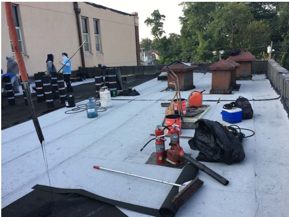
August 2018: Belleville ES #9 – Cap Sheet being installed on low Roof A
