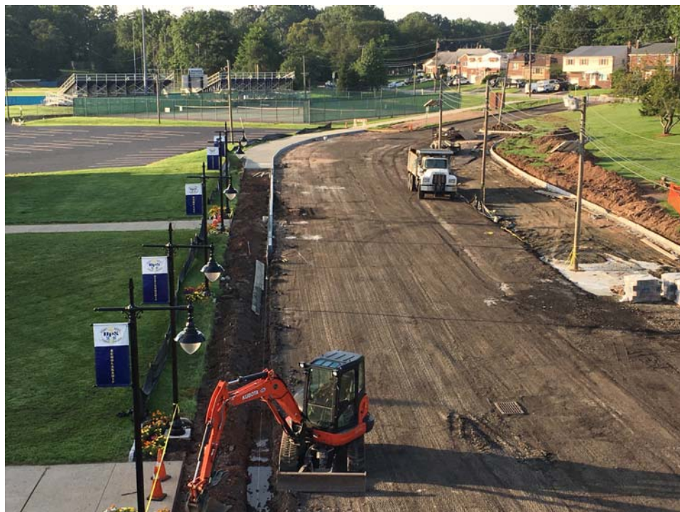
August 2018: Belleville HS – Ongoing construction activities at front “U” drive.
