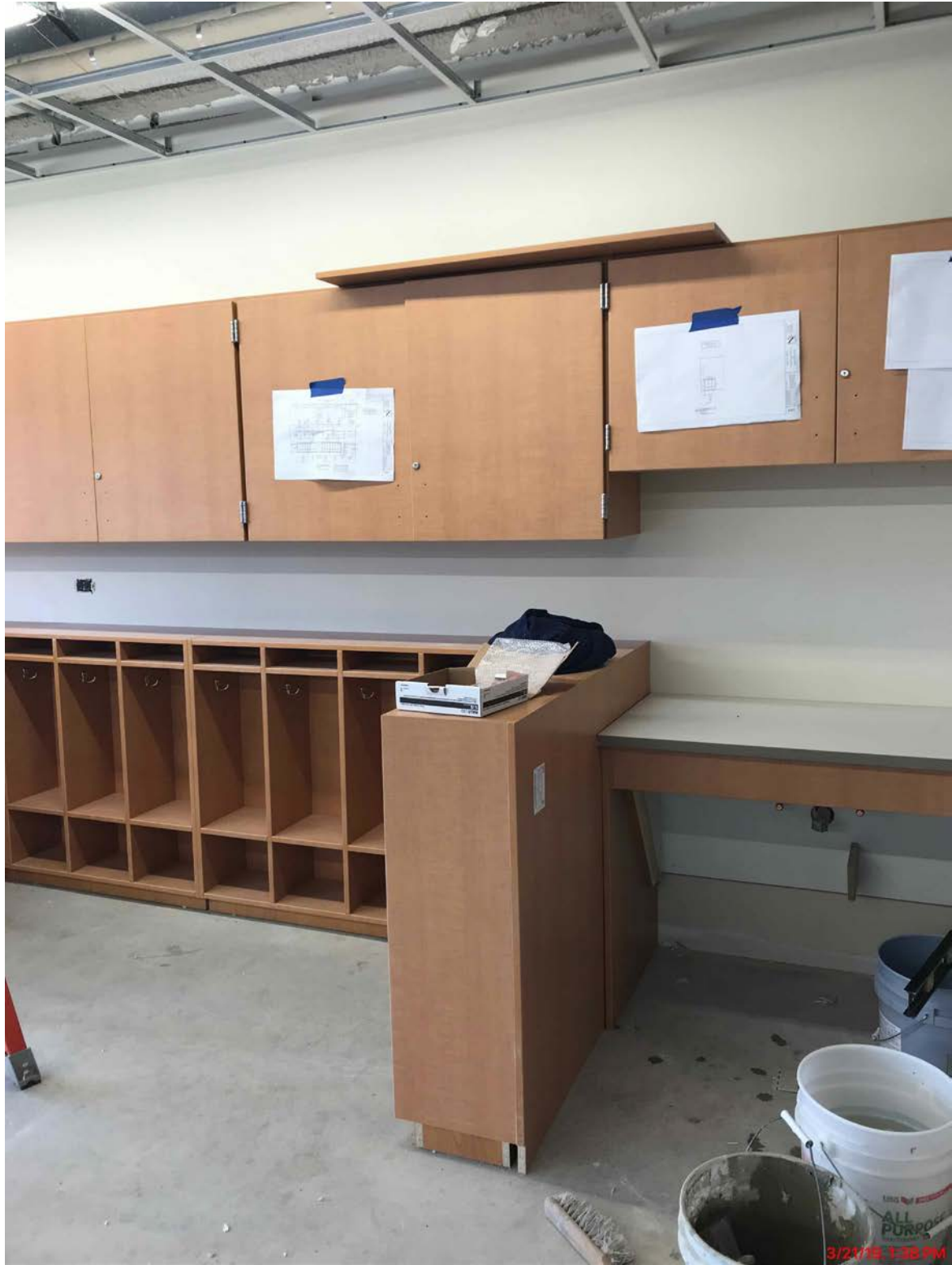
Cabinetry Installed in Eight Elementary Classrooms
