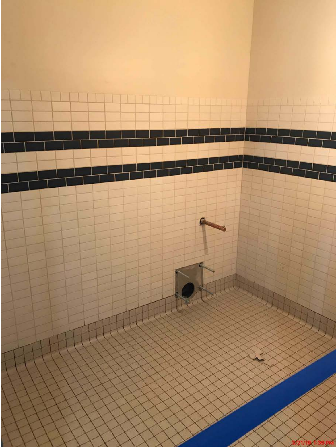
Bathroom Tile Installed in Eight Elementary Classrooms
