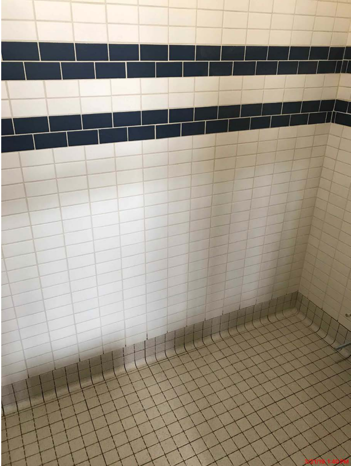
Bathroom Tile Installed in Eight Elementary Classrooms
