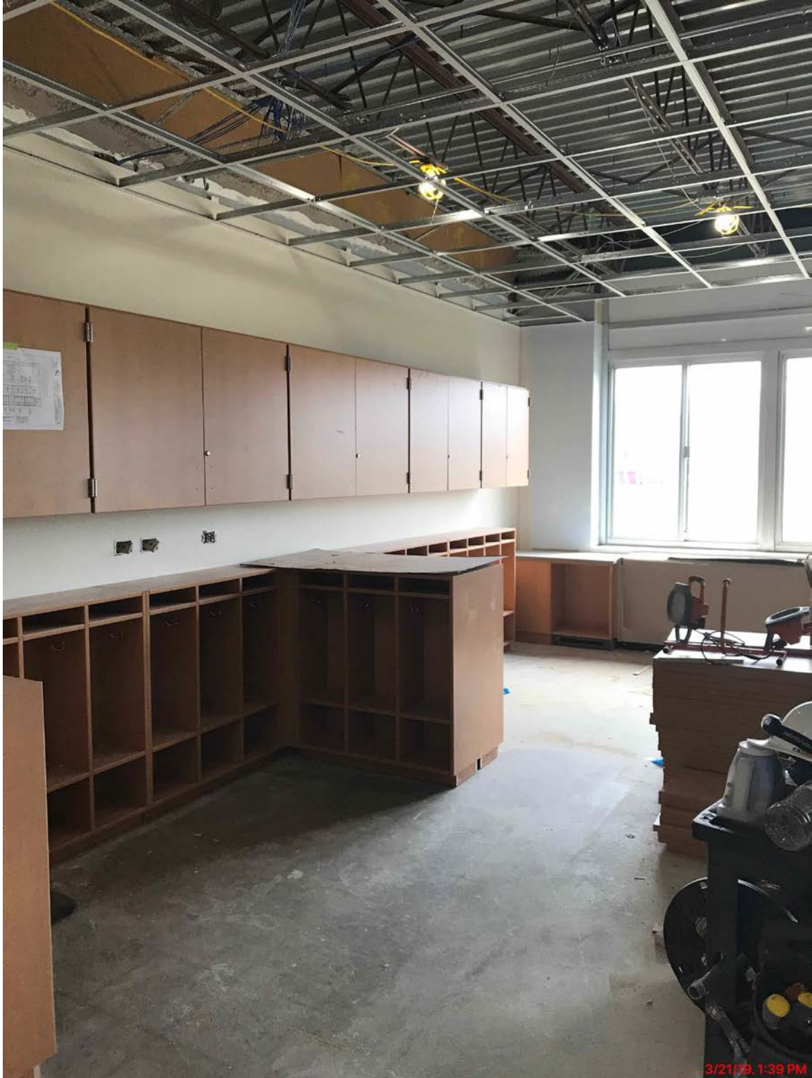
Cabinetry Installed Eight Elementary Classrooms
