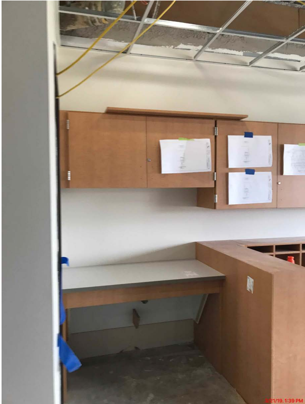
Cabinetry Installed in Eight Elementary Classrooms
