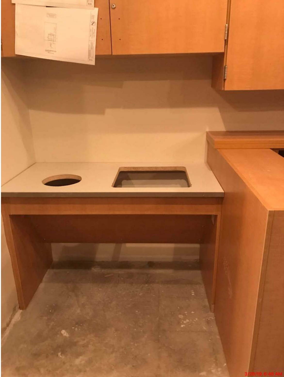
Accessible Sink and Bubbler Installed in Eight Elementary Classrooms
