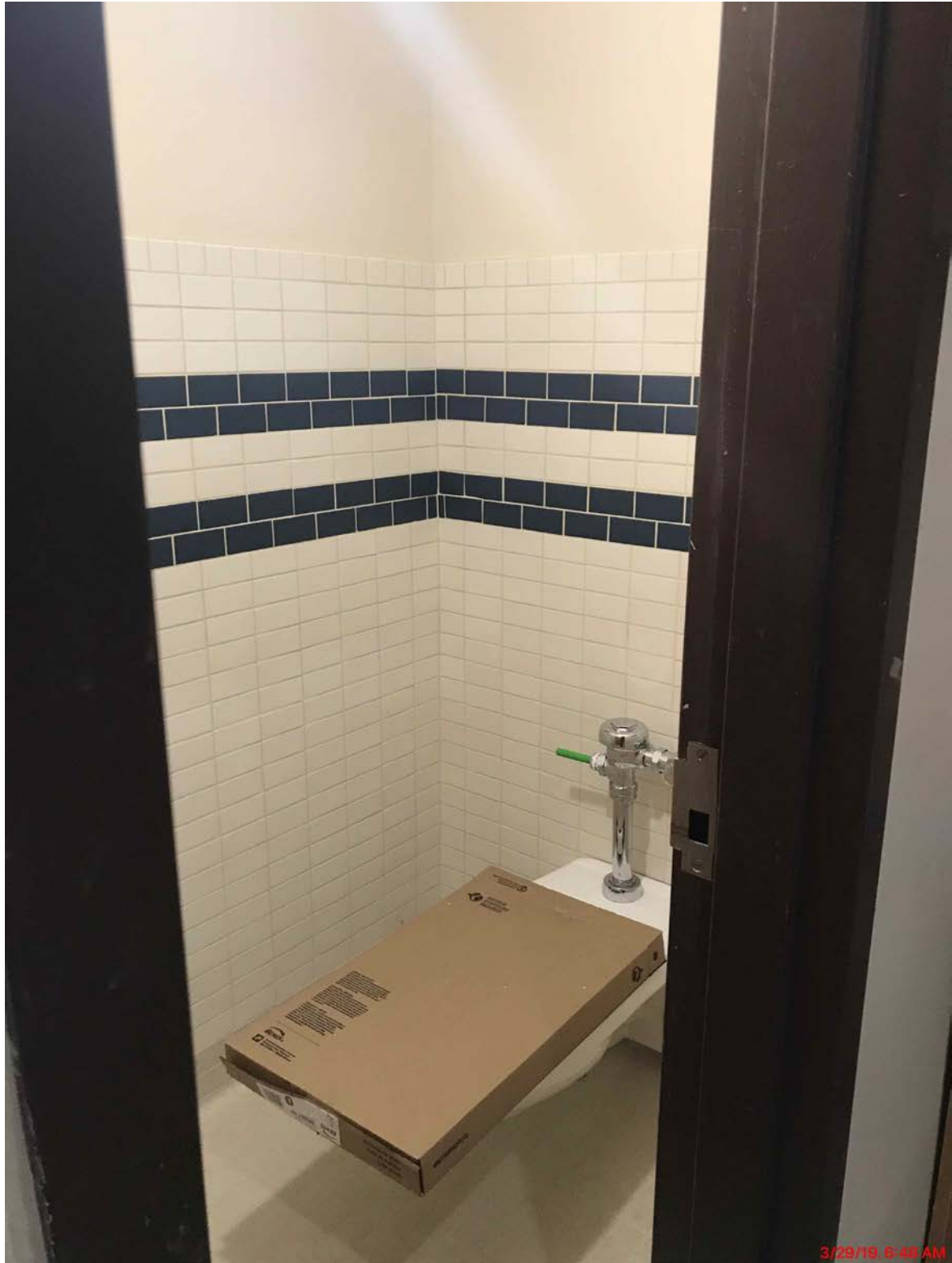
Tiling Installed in Eight Elementary Classrooms
