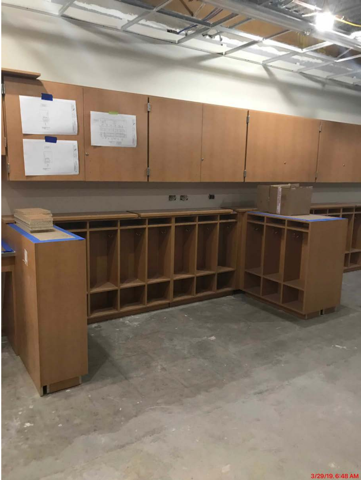
Cubbies Installed Eight Elementary Classrooms
