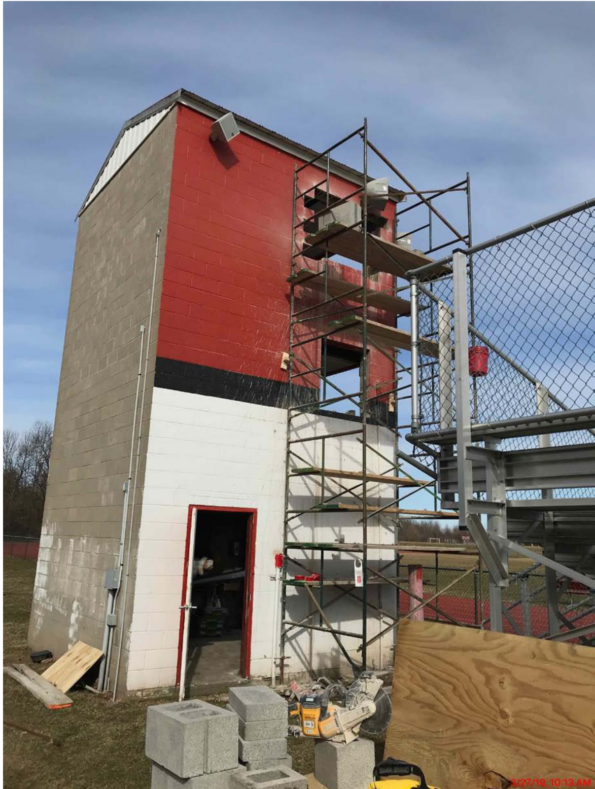
Second Egress Installed for Second and Third Floor of Football Tower
