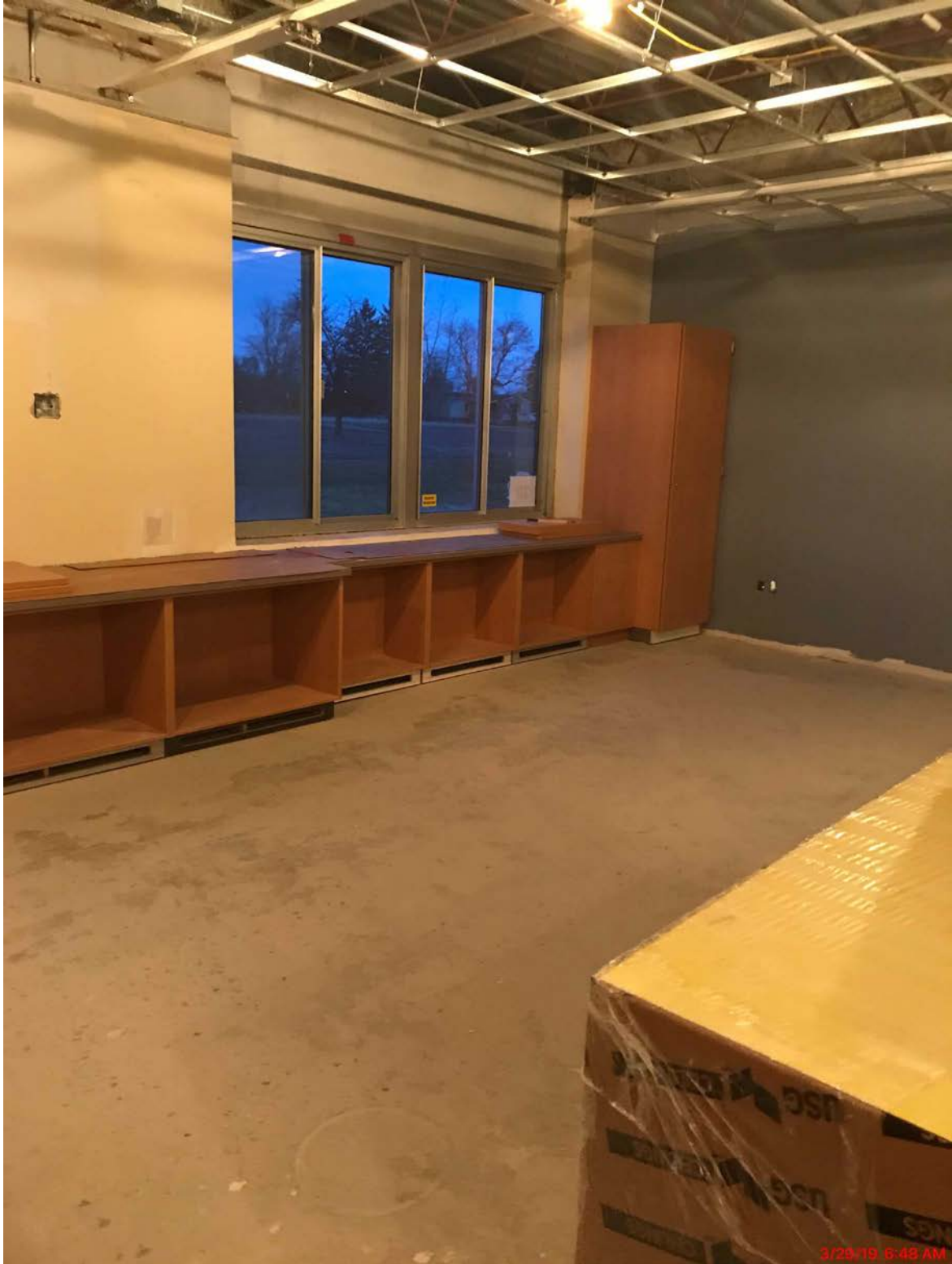
Cabinetry Installed in Eight Elementary Classrooms
