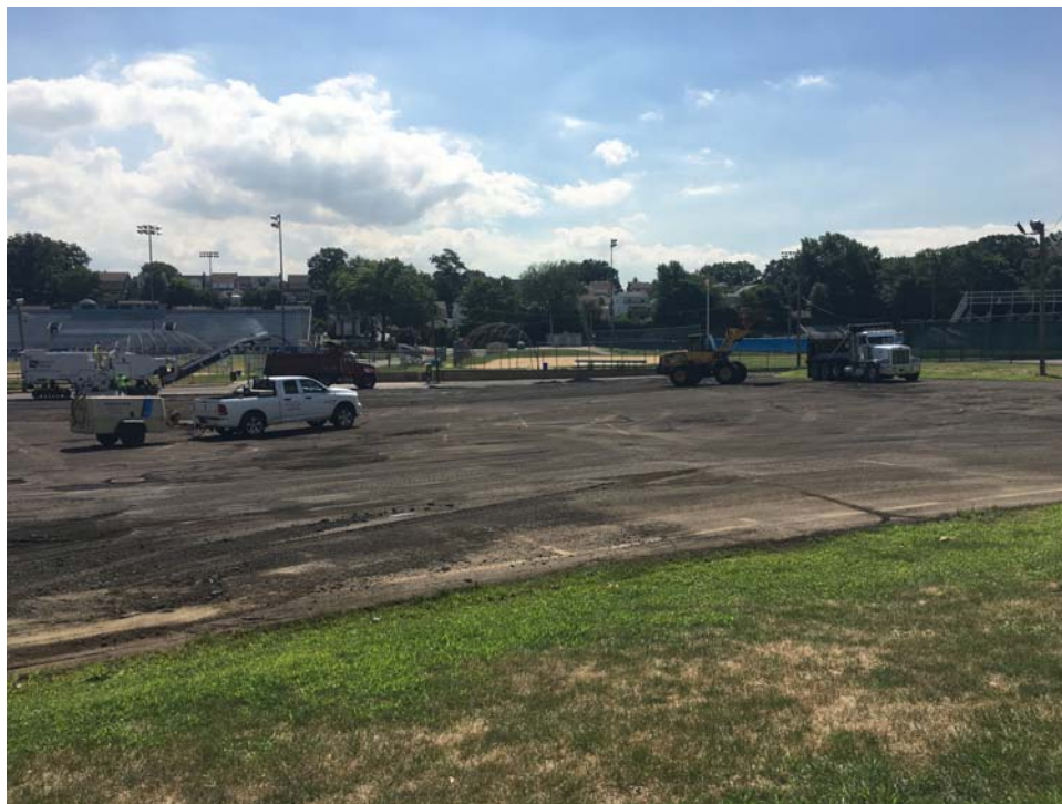
July 2018: Belleville HS – The commencement of parking lot milling activities.
