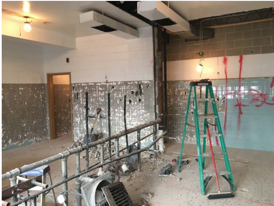
July 2018: Belleville HS –Ongoing demolition in high school 1 st floor student toilets #137 & #138.
