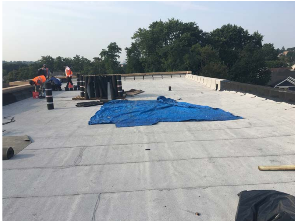
August 2018: Belleville ES #9 – Parapet flashing being installed at high Roof B.
