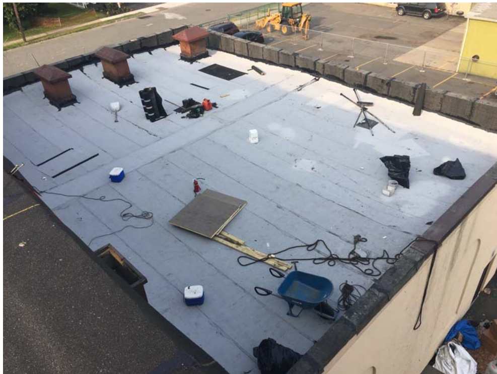
August 2018: Belleville ES #9 – Completed Cap Sheet installation on low Roof A
