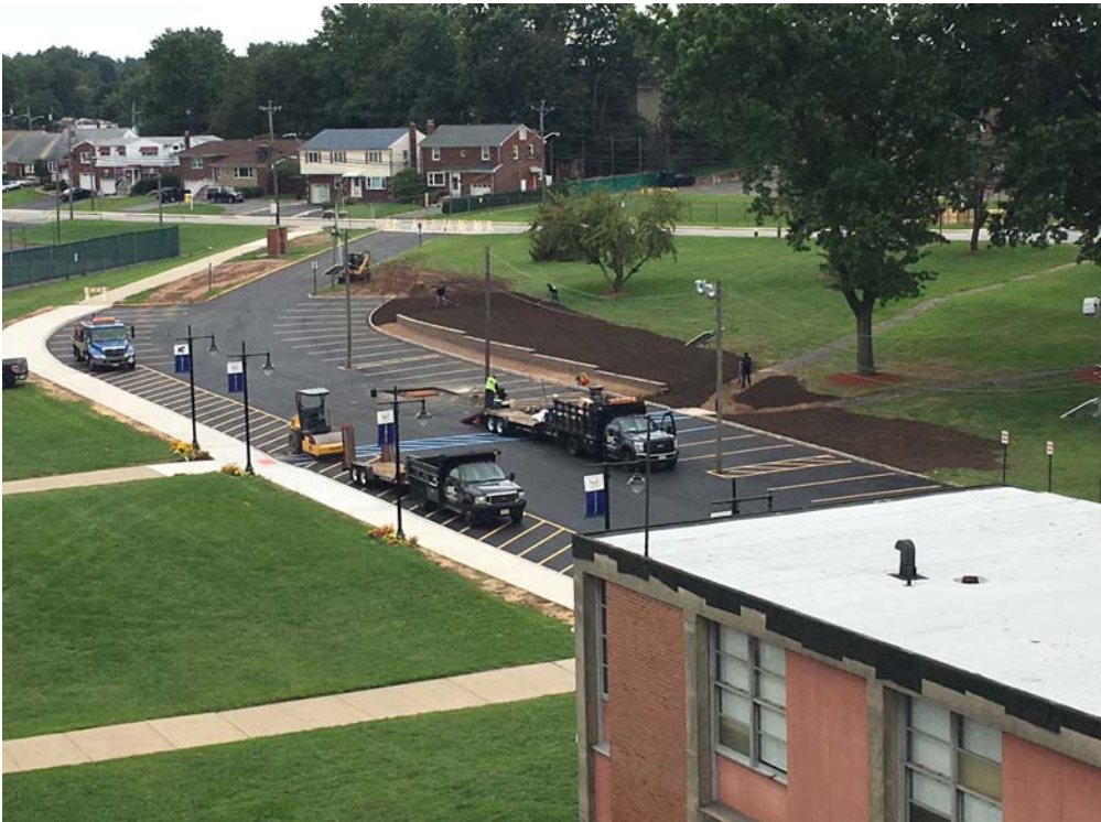
August 2018: Belleville HS – Top soil being installed at new retaining wall.
