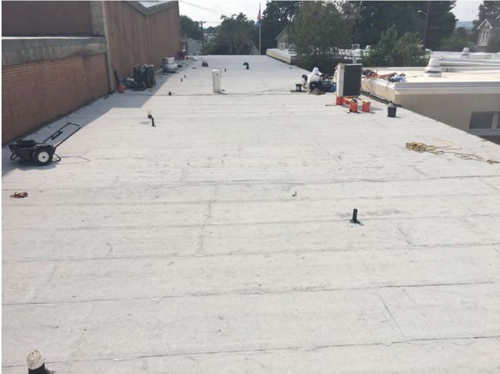
August 2018: Belleville HS – Completed Cap Sheet installation at Roof D.
