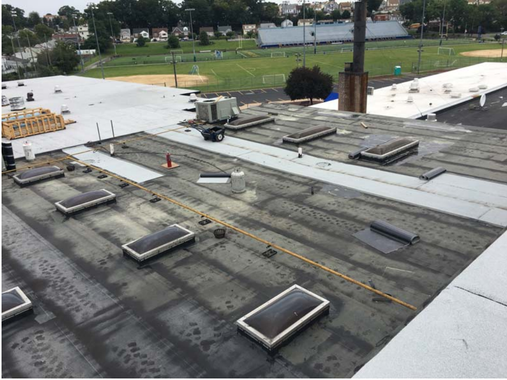
August 2018: Belleville HS – Cap sheet installation commencing on Roof B.
