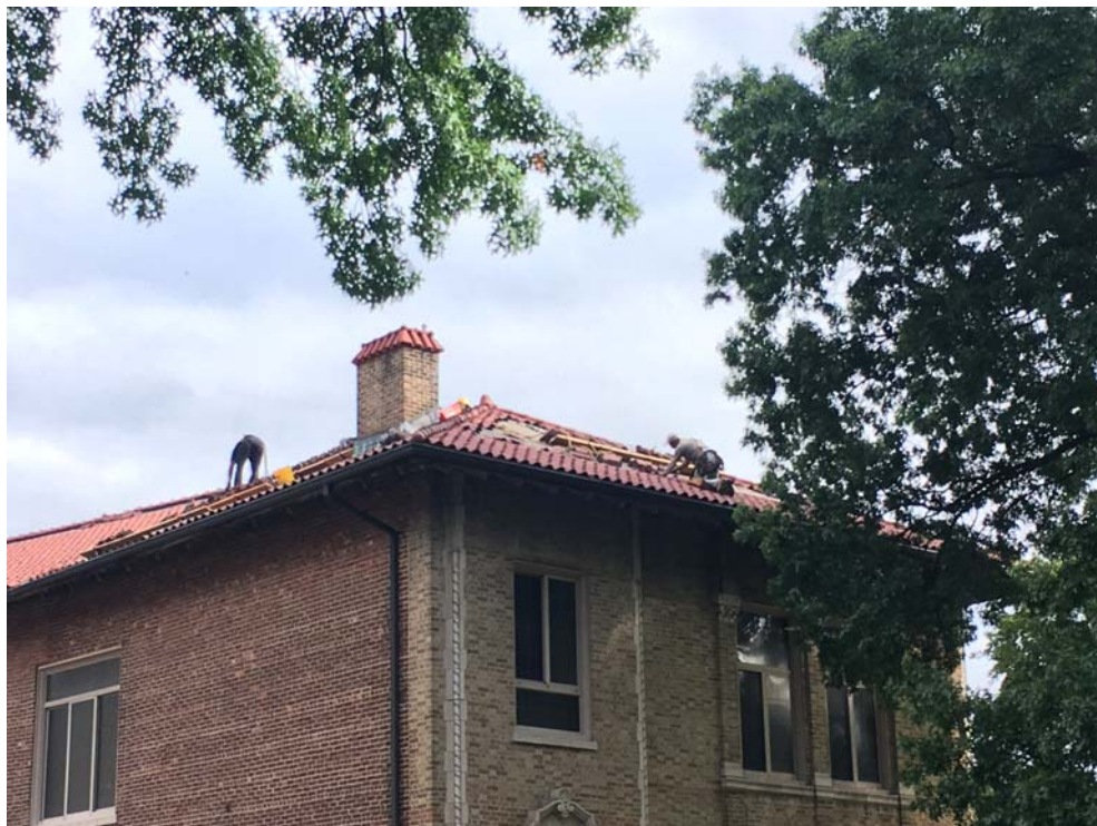
August 2018: Belleville ES #10 – Tile reinstatement following deck repairs & underlayment installation.
