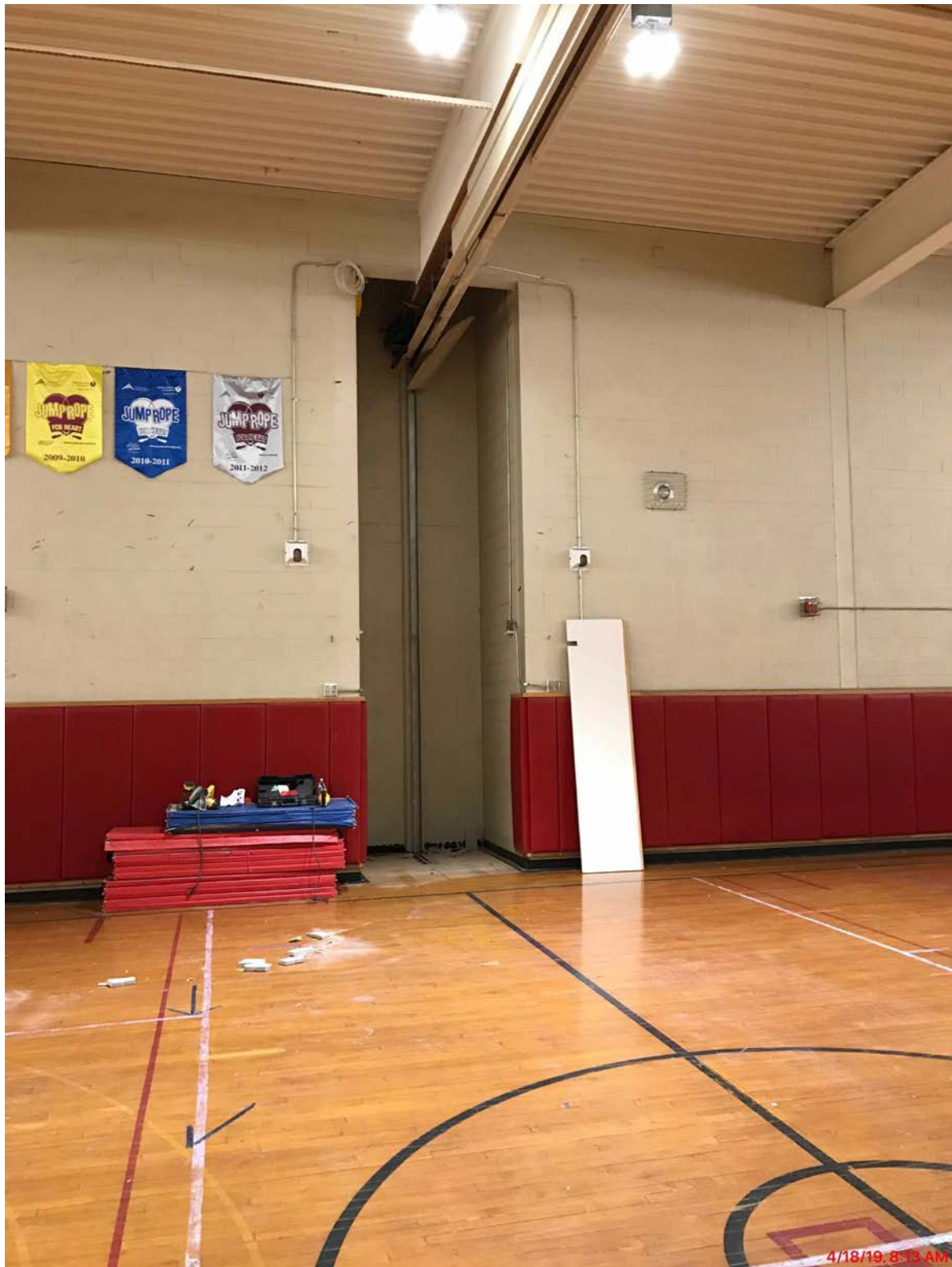
Removal of Dividing Door Elementary Gym
