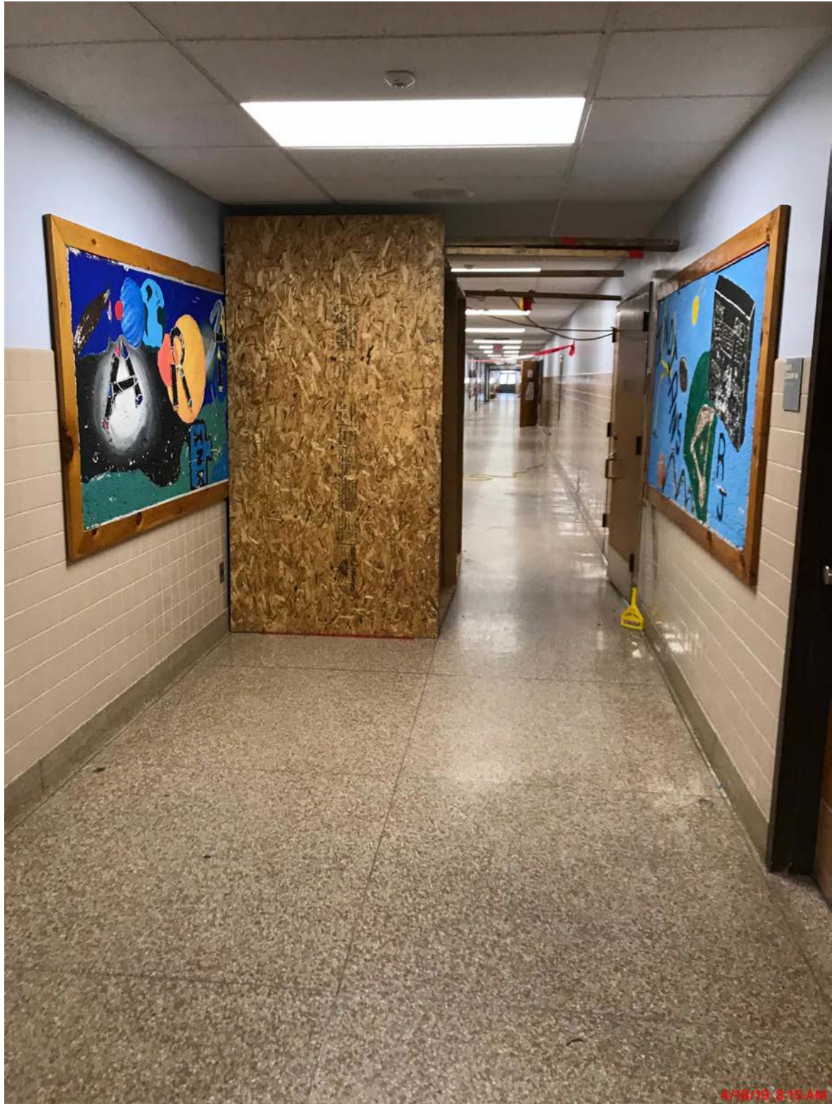
Abatement of Elementary Art Room over Spring Break
