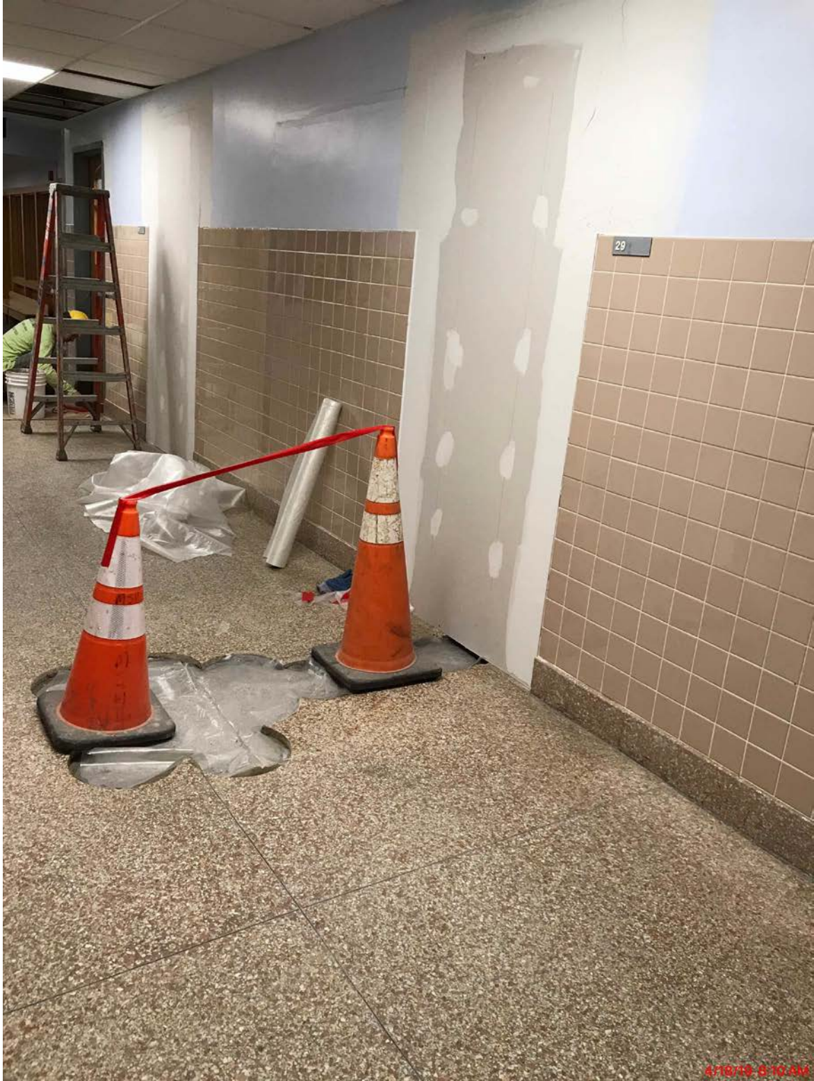
Plumbing Installed for New District Office
