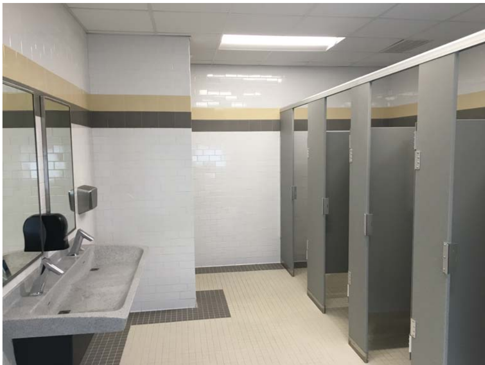
September 2018: Belleville HS - 1 st floor Girls' Toilet completed and ready for use.
