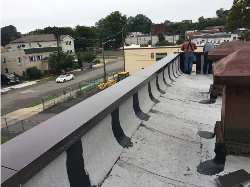
September 2018: Belleville ES #9 – Copings being installed at low Roof A.
