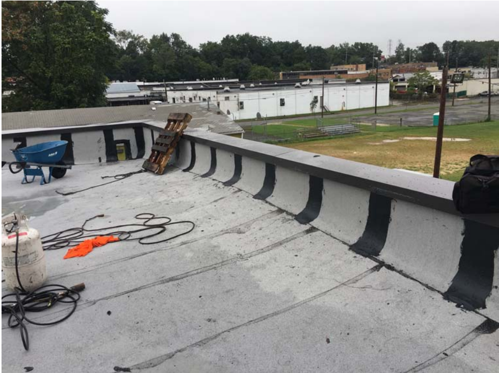
September 2018: Belleville ES #9 – Perimeter trims (copings) delivered and hoisted up to roof.
