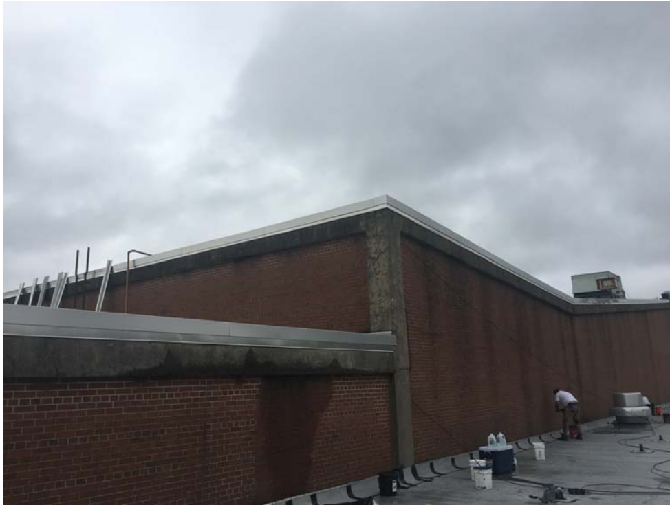
September 2018: Belleville HS – Completed perimeter trim installation at Roofs B & C.
