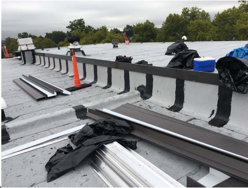
September 2018: Belleville ES #3 – Metal perimeter trims (fascia extensions) installation in progress.
