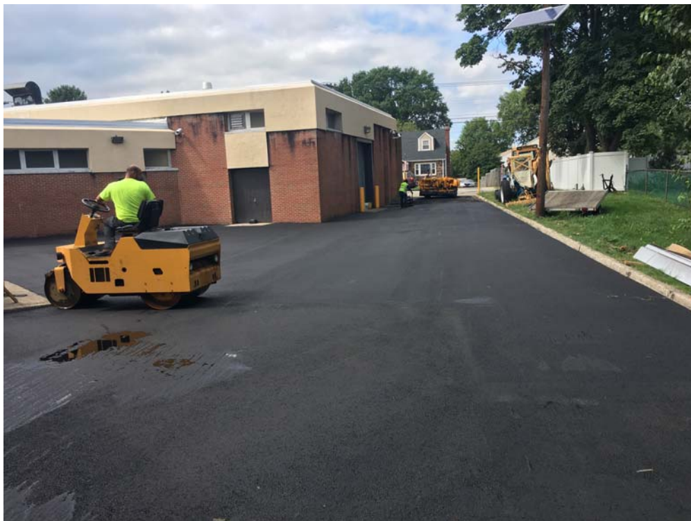
September 2018: Belleville HS – Paving at drive to Door #7 completed.
