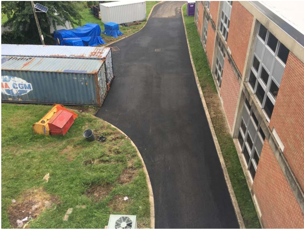
September 2018: Belleville HS – Paving at rear drive completed.
