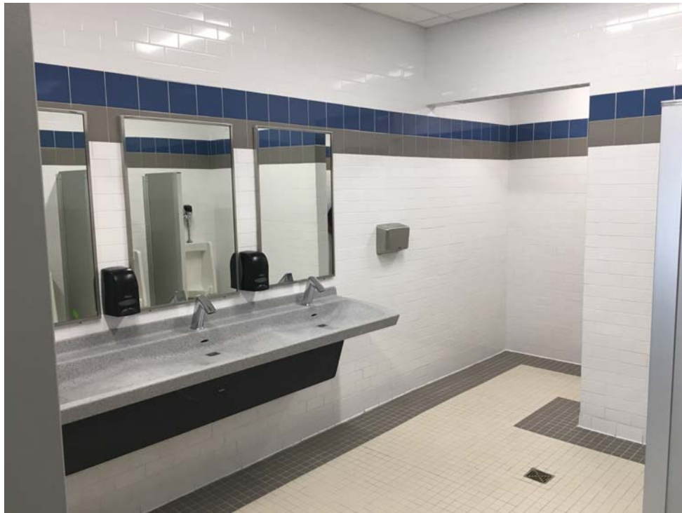
September 2018: Belleville HS -1 st floor Boys' Toilet completed and ready for use.
