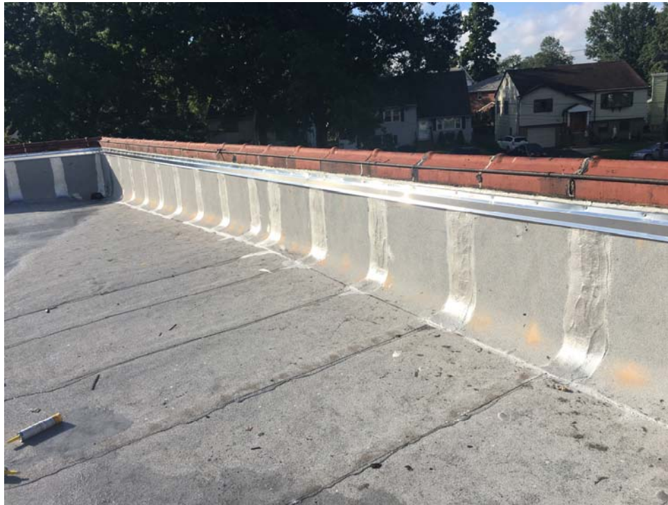
September 2018: Belleville ES #10 – Metal counter-flashings installation completed.
