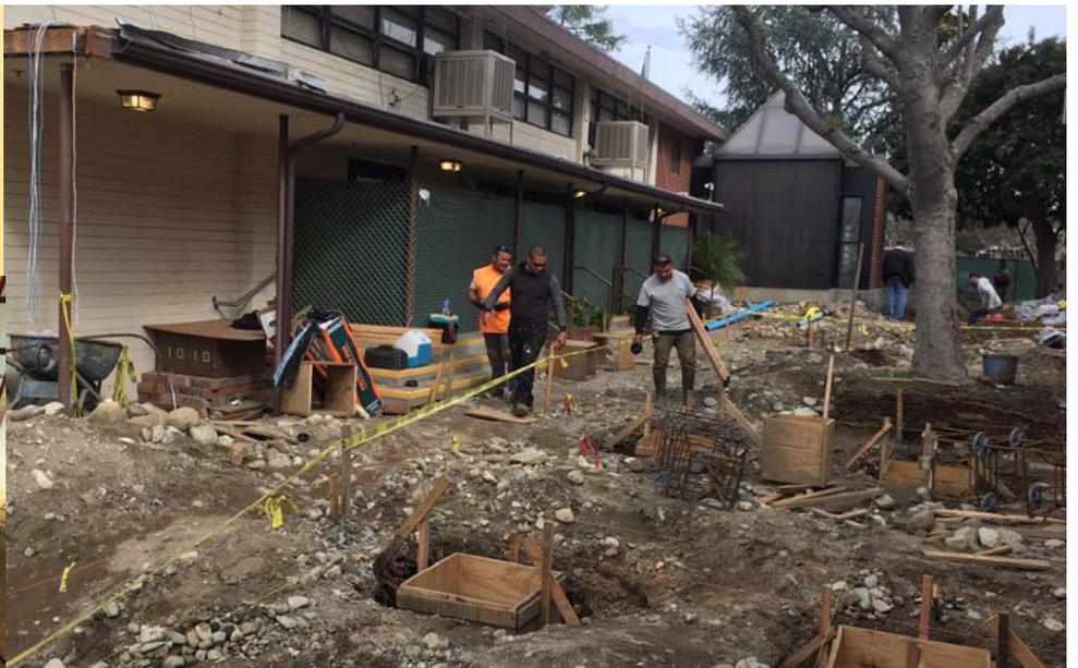
Current projects include pouring footings for new canopy and trellises, installing the new roof, rough electrical installation, framing new restrooms, rough HVAC, rough plumbing and electrical for the new baptismal font, and digging footings and installing steel for the vestibule.
