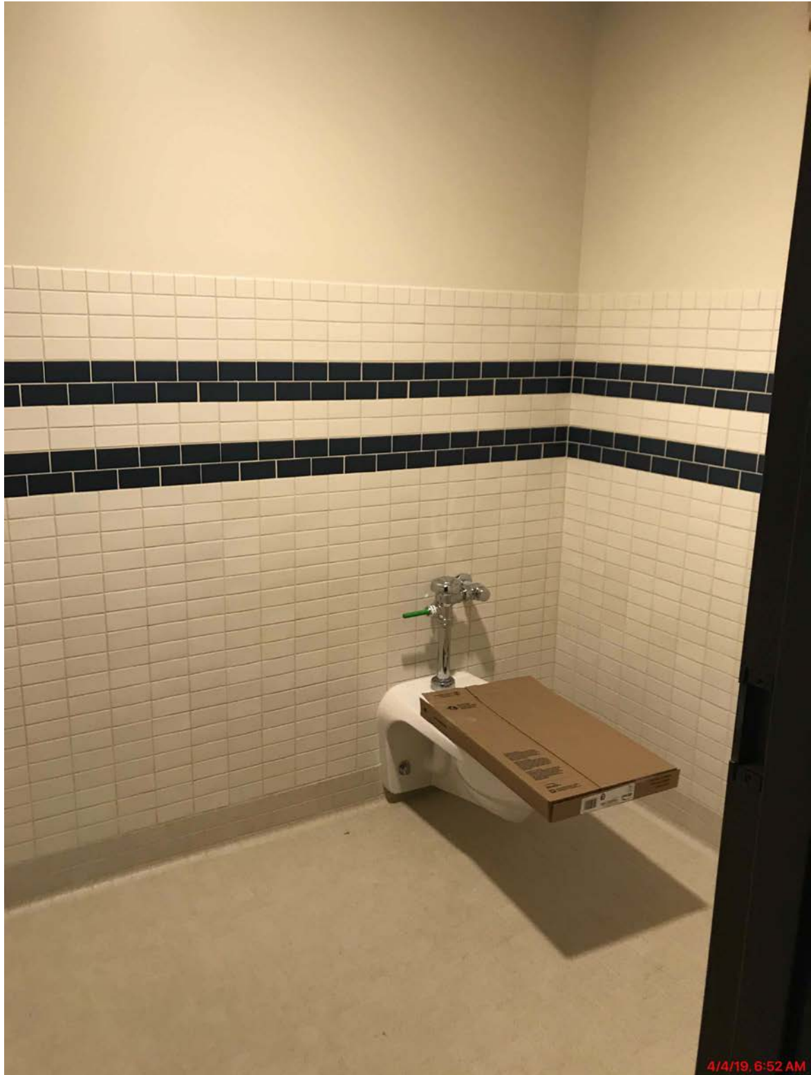
Tiling and Fixtures Installed in New Bathroom by Elementary Gym
