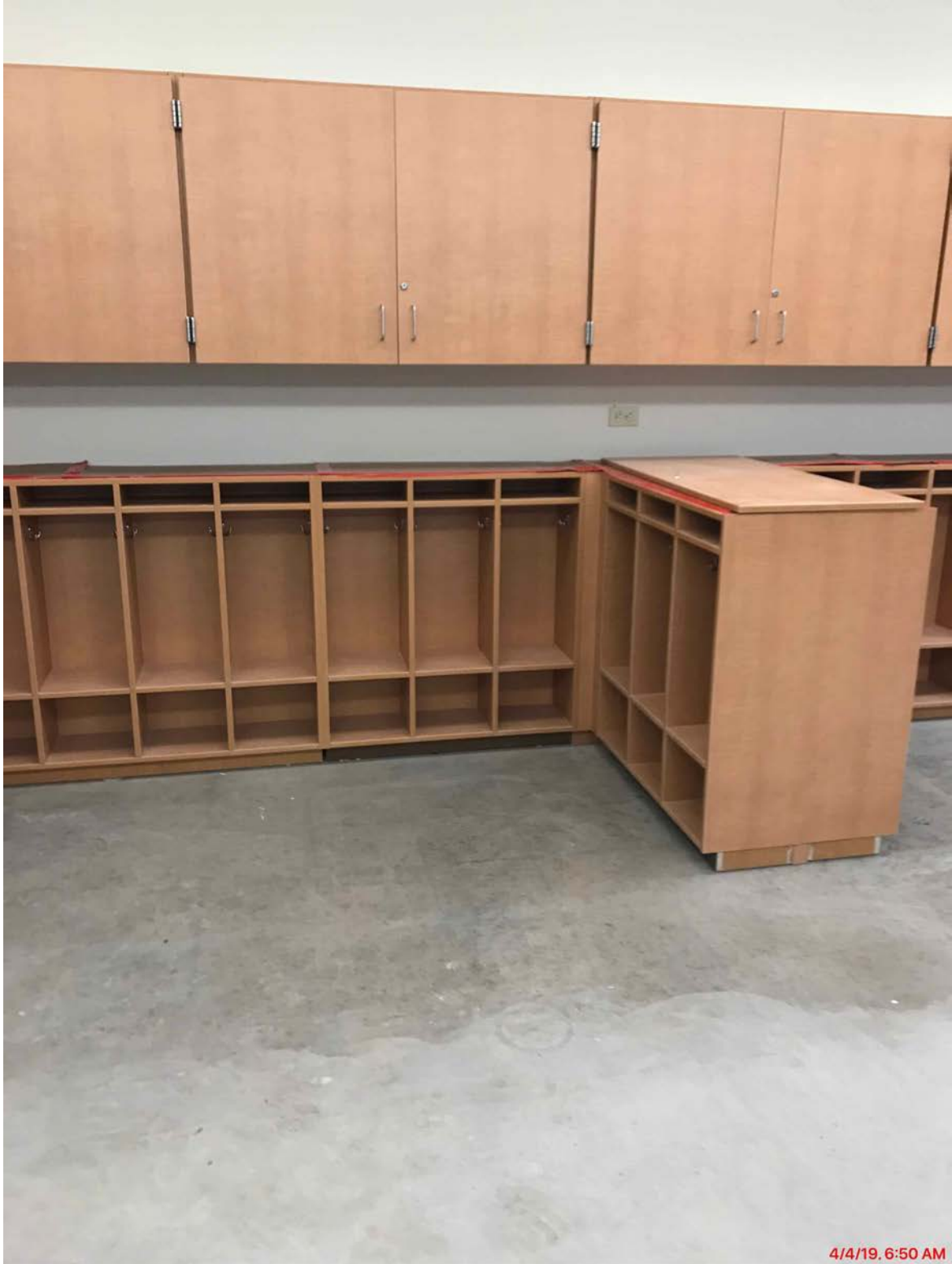
Cubbies Continue to be Installed in Eight Elementary Classrooms
