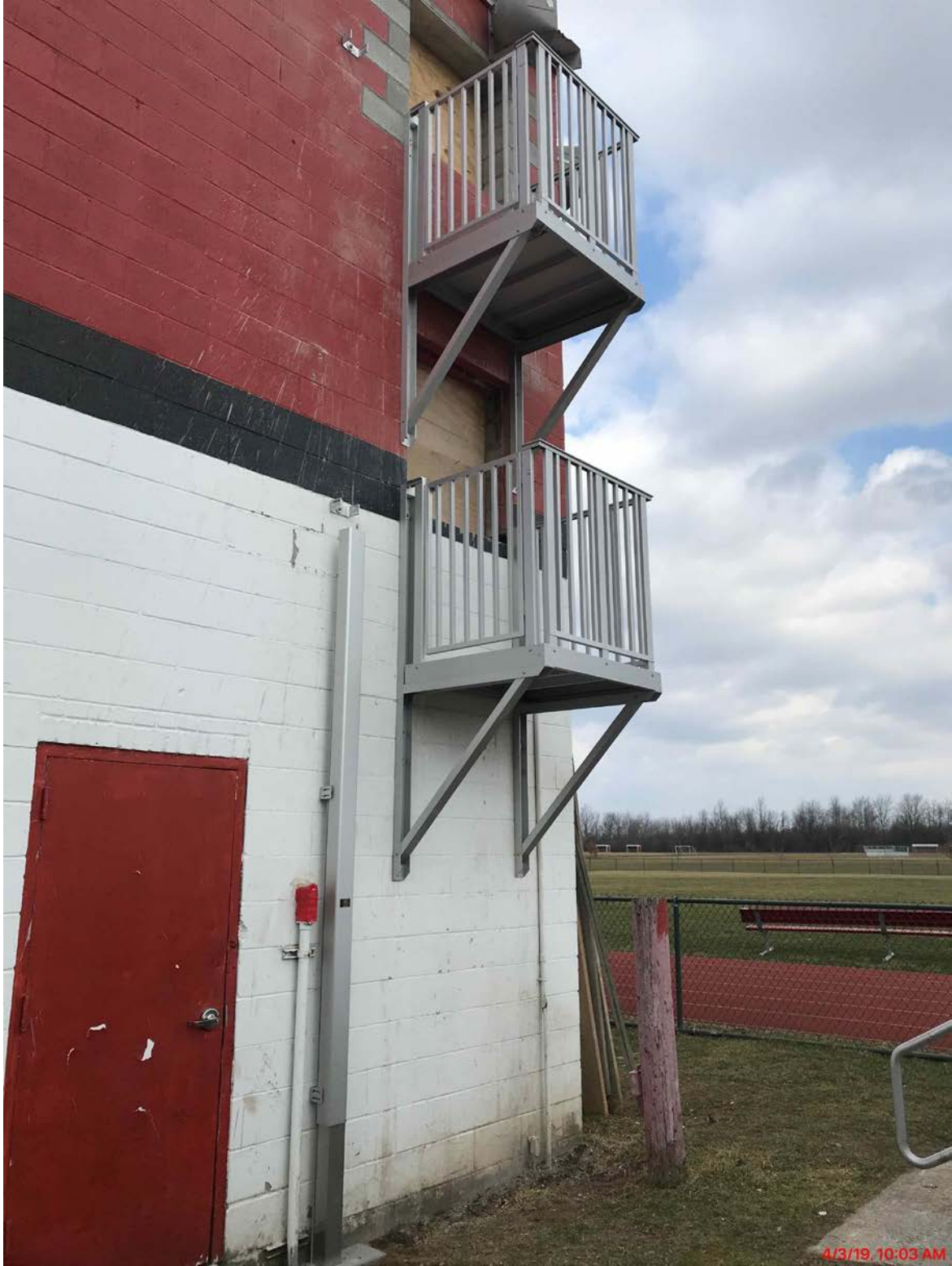
Work Continues on Second Egress for Tower
