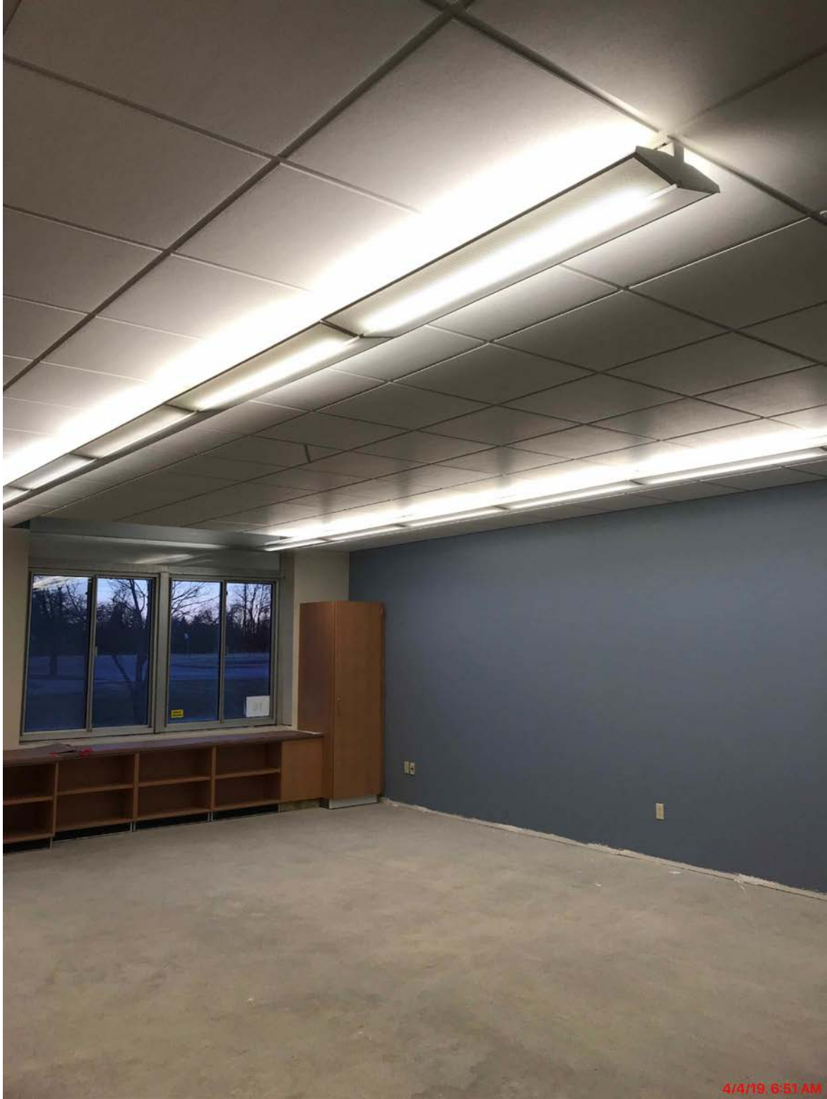
Ceiling Tiles and Lights Installed in Eight Elementary Classroom
