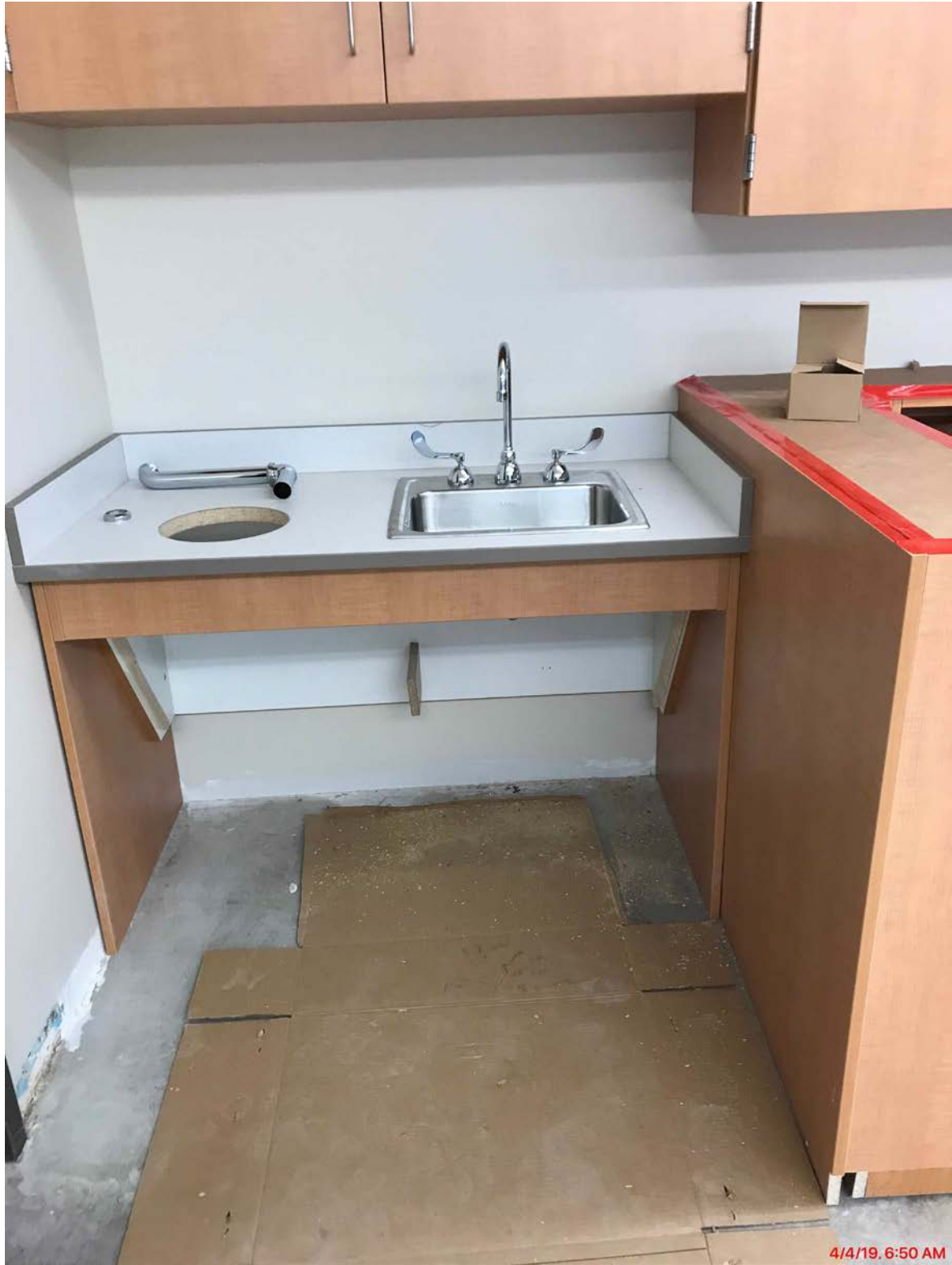
Sinks Installed in Eight Elementary Classrooms
