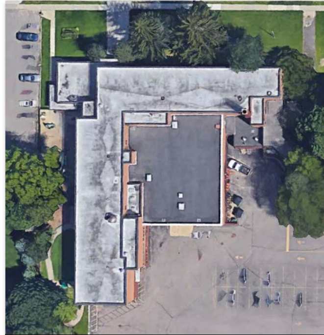
501 West Main Street - Demolition Site
