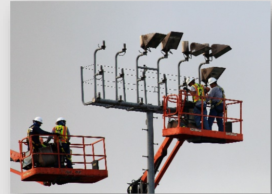
Out with the Old, In with the New Dark Sky Friendly Lights at Texan Stadium
