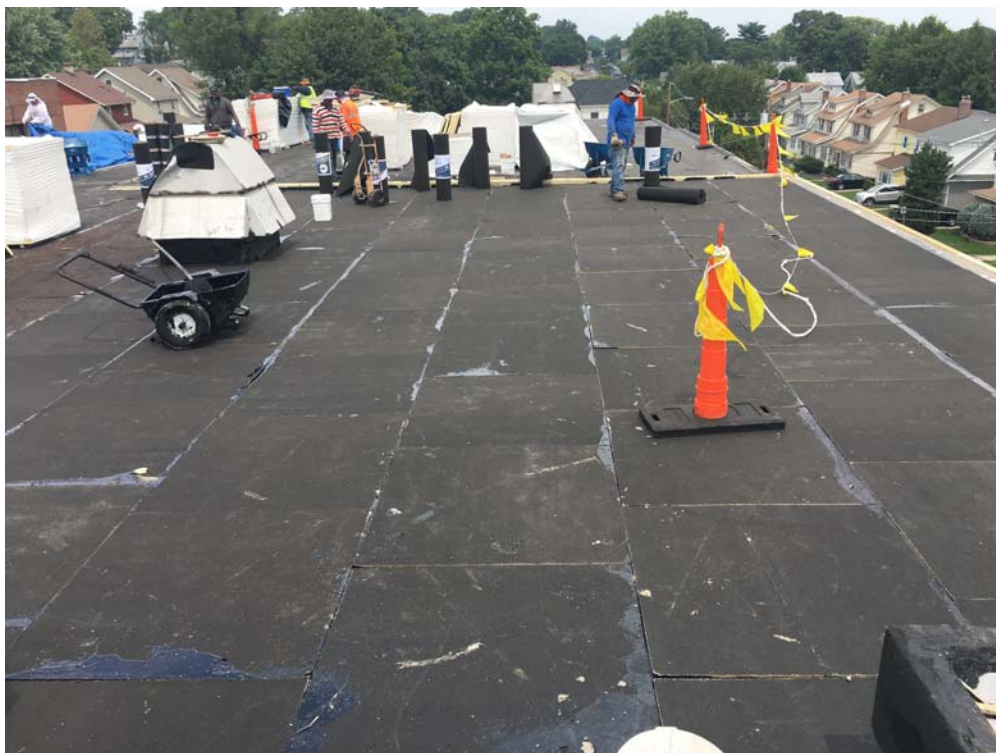
July 2018: Belleville ES #3– Cap Sheet substantially completed at Roof B.
