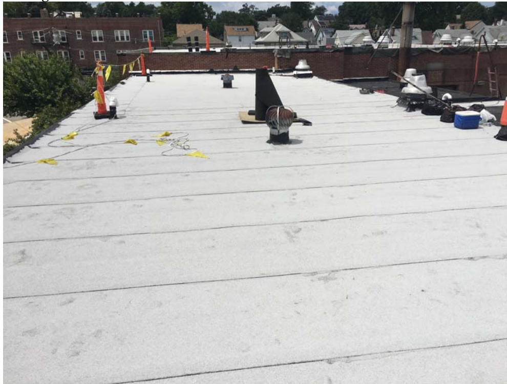
July 2018: Belleville ES #3– Cap Sheet substantially completed at Roof B.
