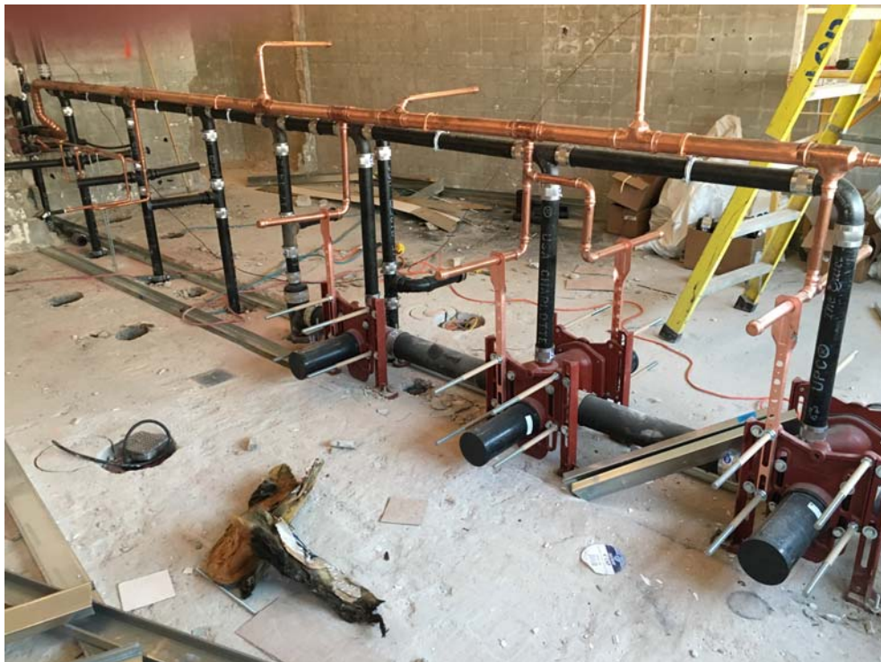
July 2018: Belleville HS – Plumbing rough-ins completed in 2 nd floor student toilets #206 & #208.
