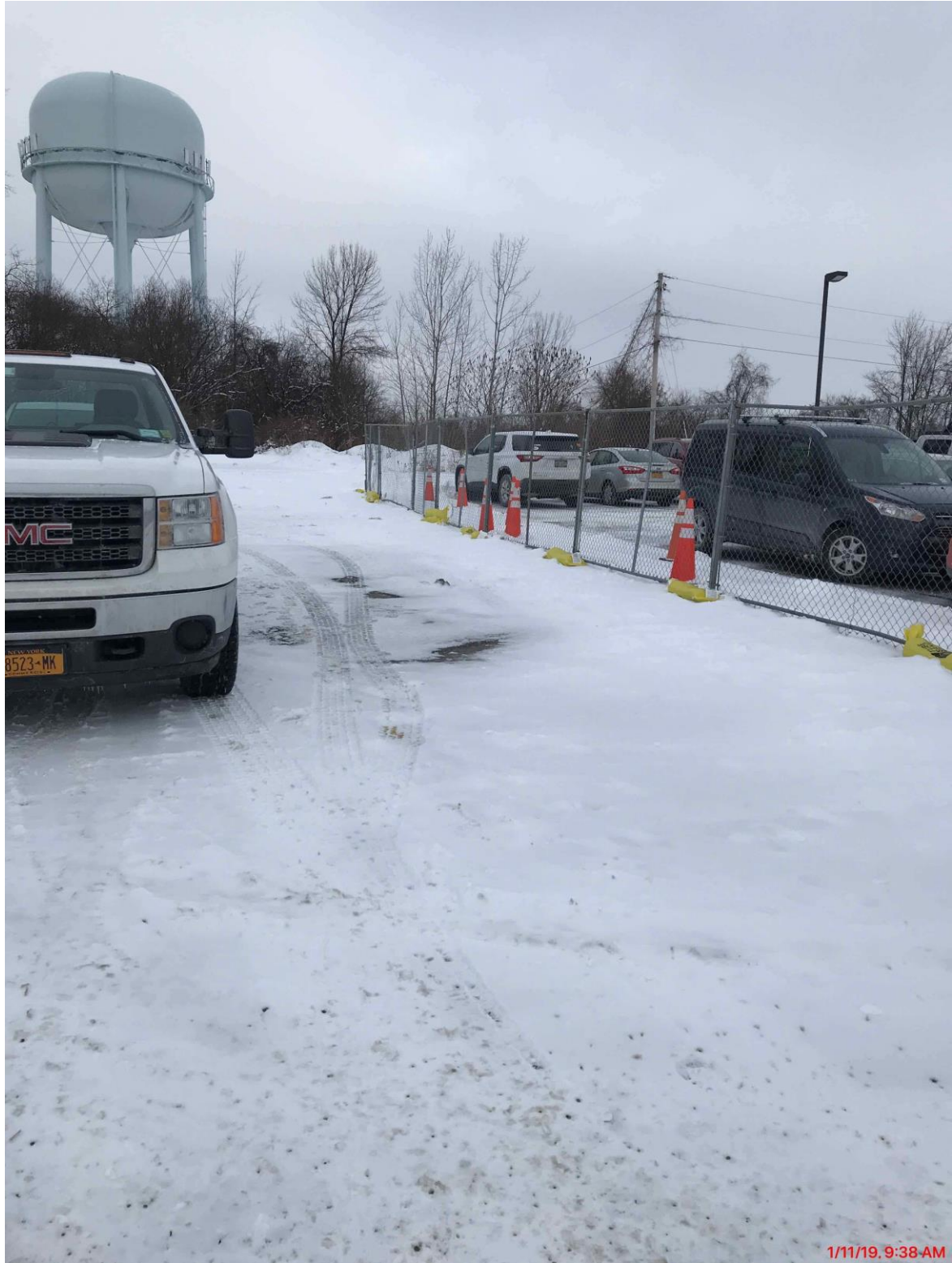
Safety Fencing Installed At Elementary School
