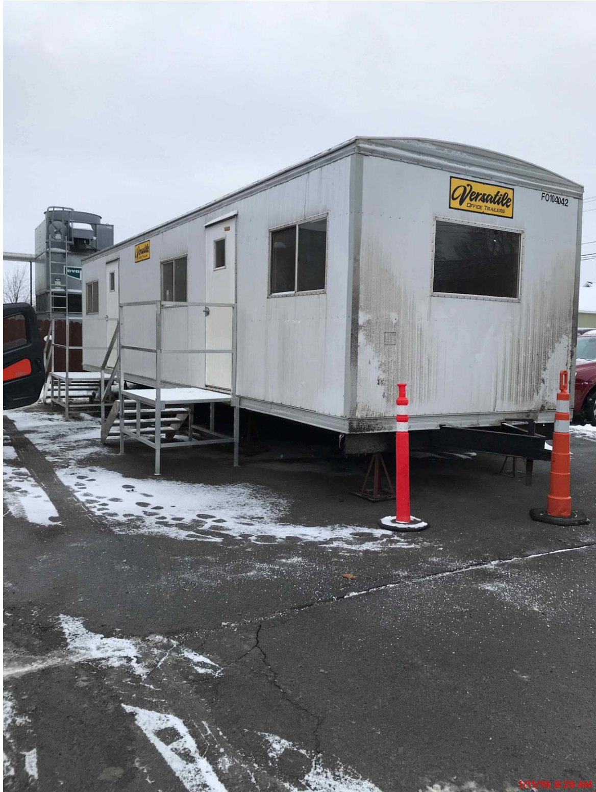
General Contractor Set UP On Site Preparing for Construction to Begin on January 14, 2019
