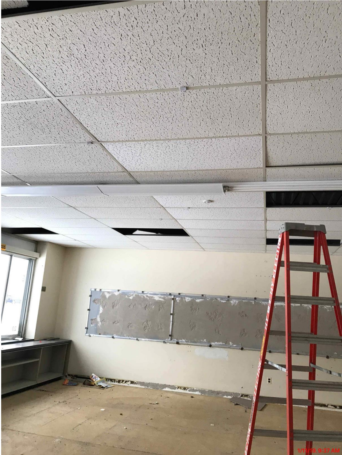
All Lights and Ceiling Tiles Removed - Eight Elementary Classrooms
