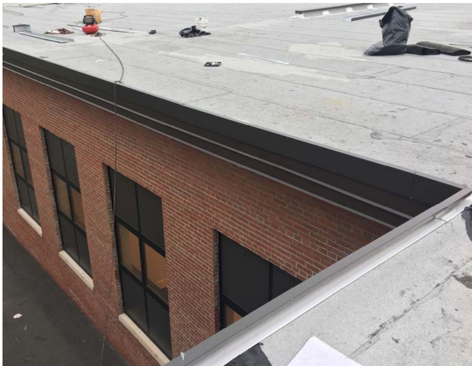
September 2018: Belleville ES #3 – Metal perimeter trims (fascia extensions) installation (Photo 2)
