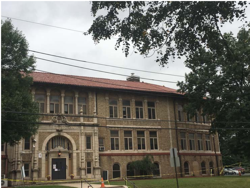
September 2018: Belleville ES #10 – Roof Tile work completed at ES #10 (Photo 2)
