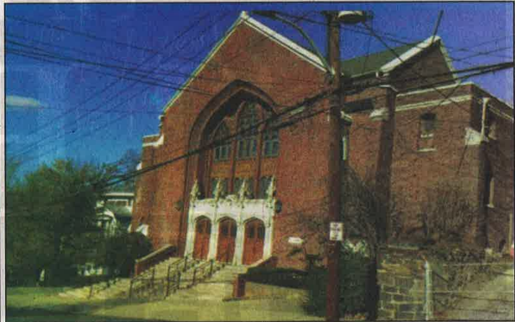
The former Our Lady of Rosary Church, the site of the new Yonkers Charter High School.
