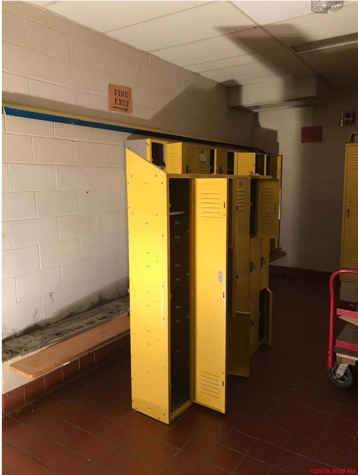
Removal of Lockers in Elementary Locker Rooms
