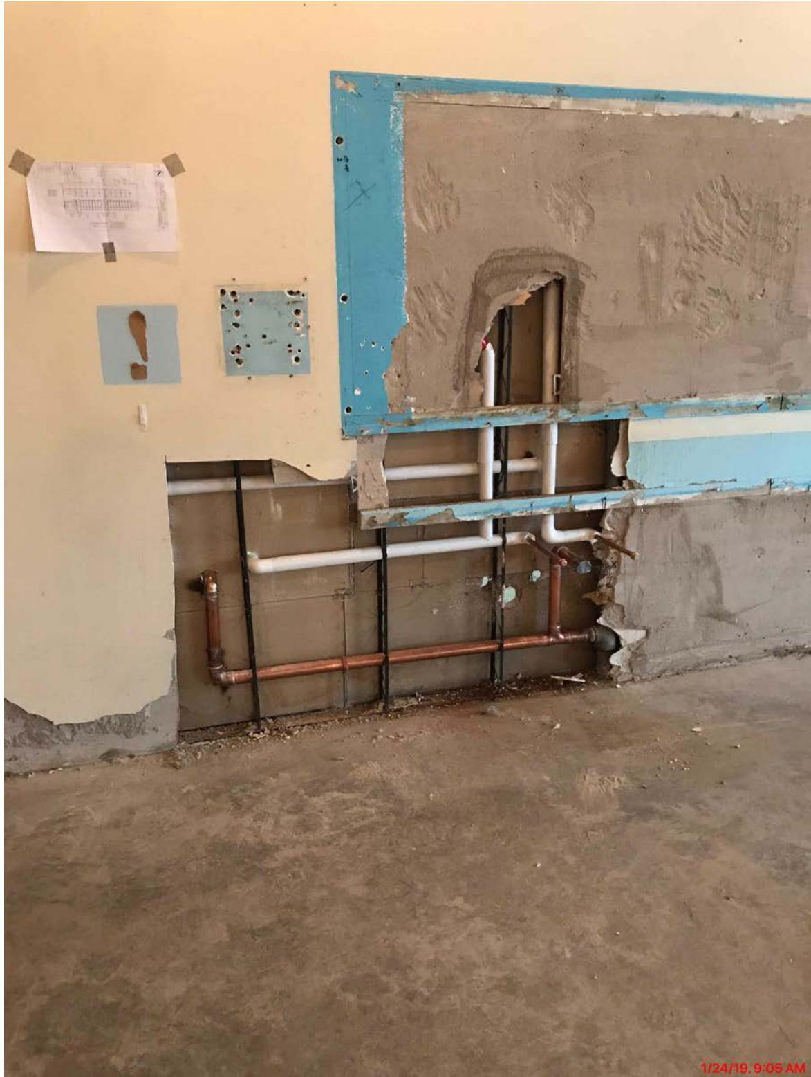
Upgrading of Plumbing Continues - Eight Elementary Classrooms
