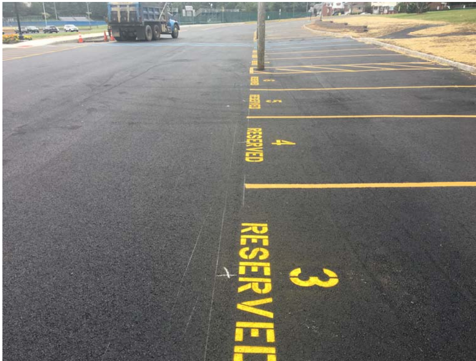
September 2018: Belleville HS – Stenciling at Front “U” drive completed.
