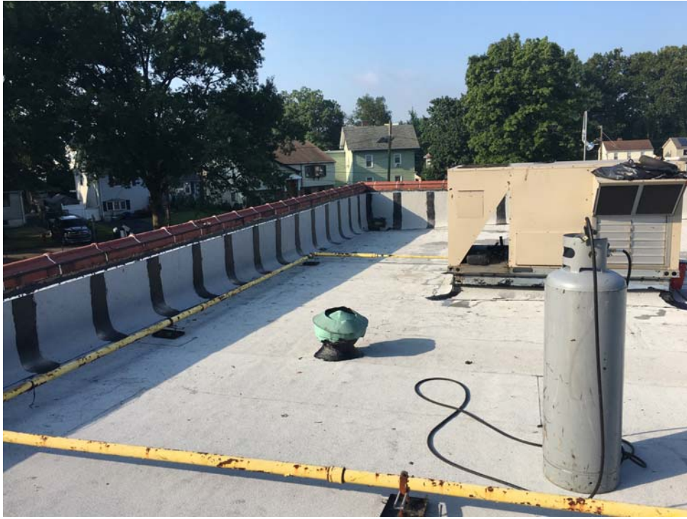
September 2018: Belleville ES #10 – Parapet flashing completed on the flat roof.
