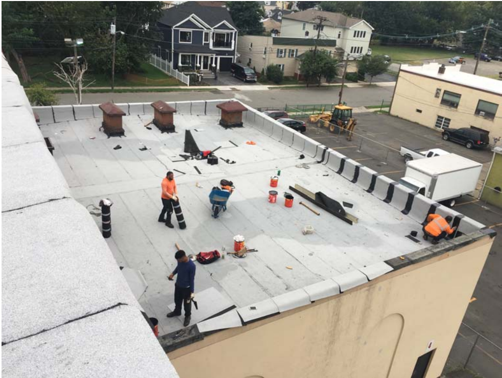
September 2018: Belleville ES #9 – Parapet flashing being completed at low Roof A.
