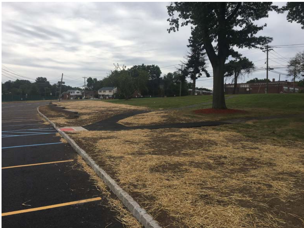
September 2018: Belleville HS – Soil stabilization completed at areas of disturbance.
