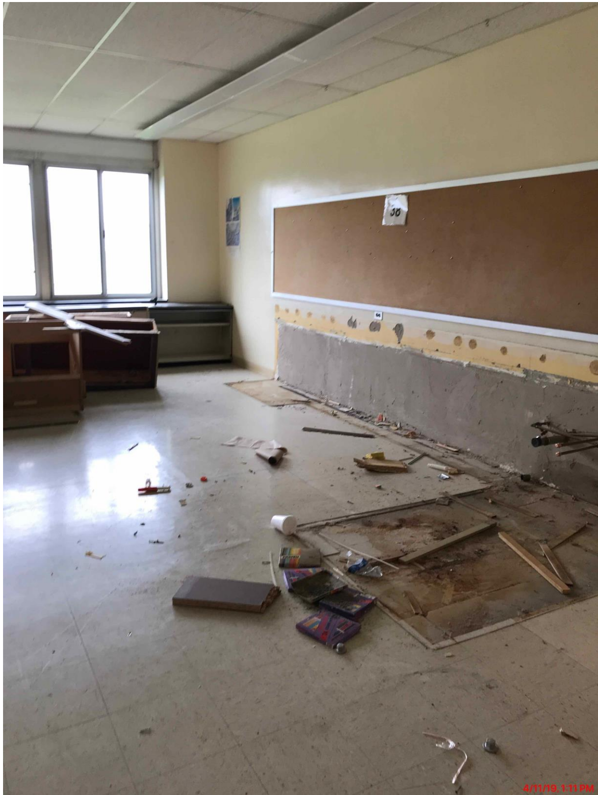
Pre Abatement Demolition in Elementary Art Room
