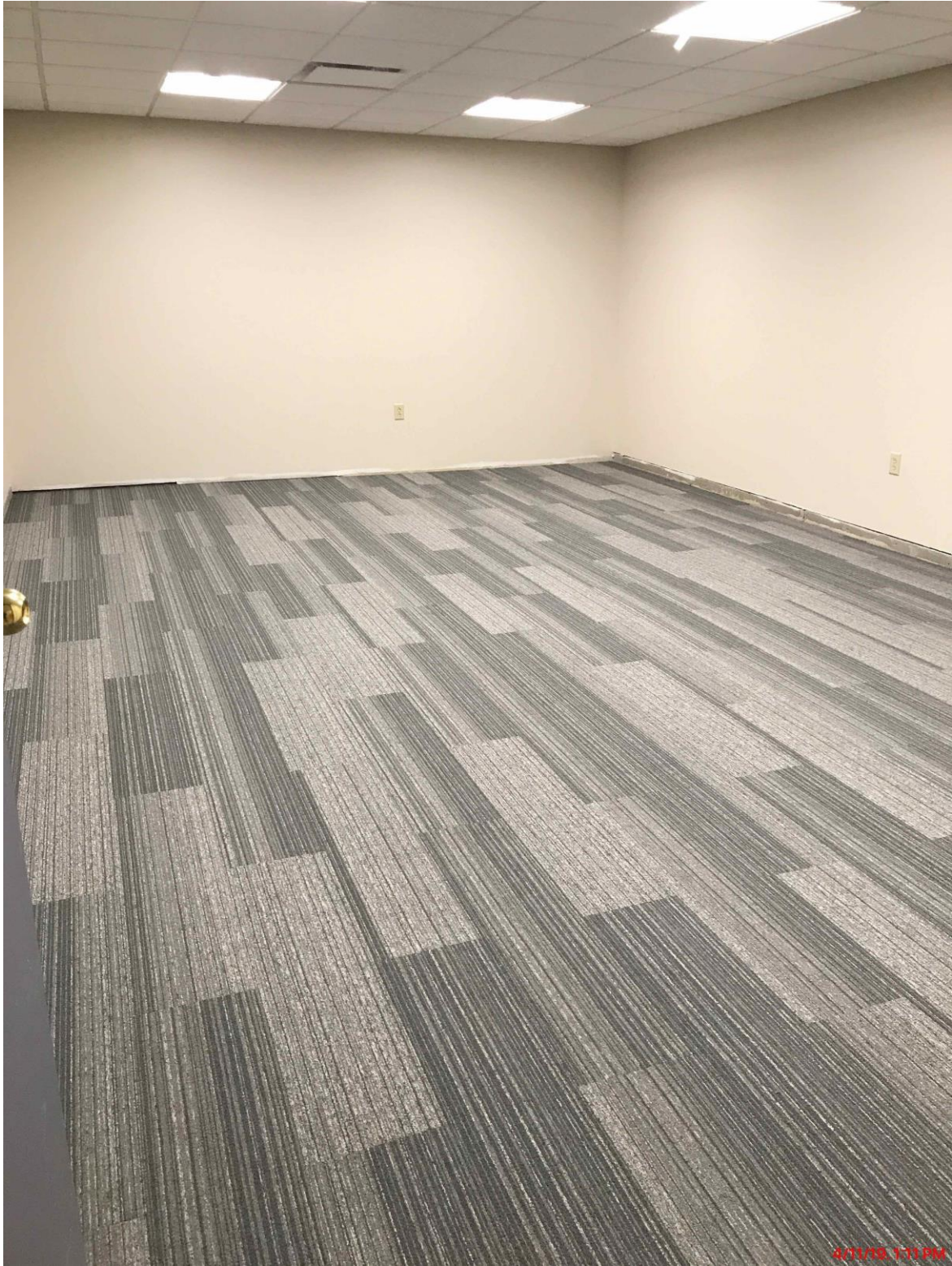
Carpet Installed in New Elementary Sensory and PT/OT Rooms
