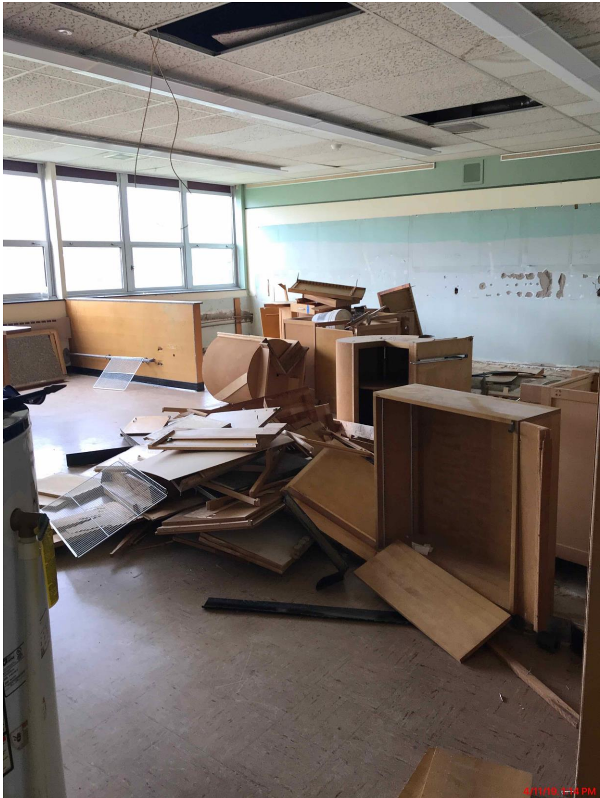
Pre Abatement Demolition in High School FACS Room
