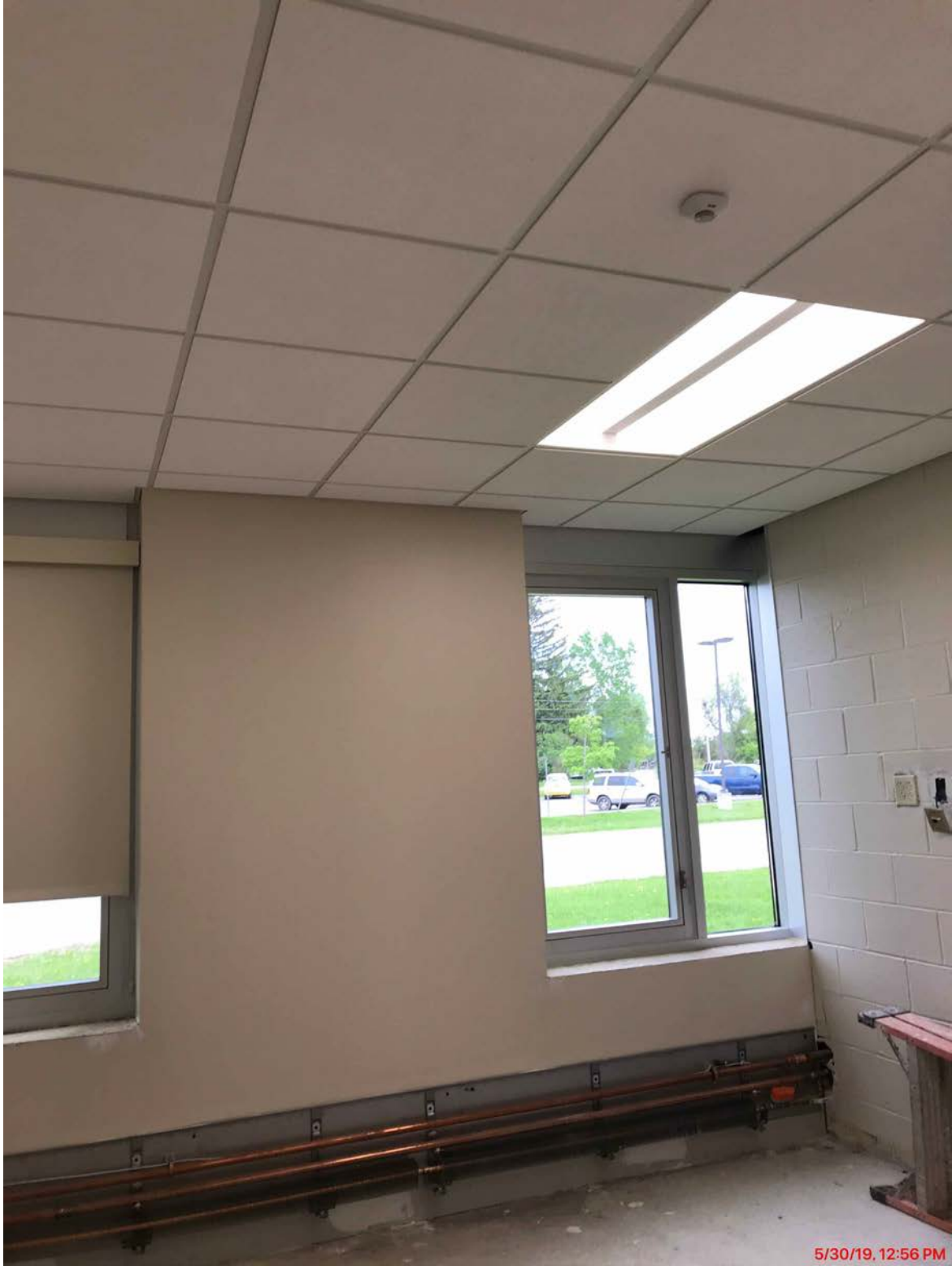
Window Installation Continues
