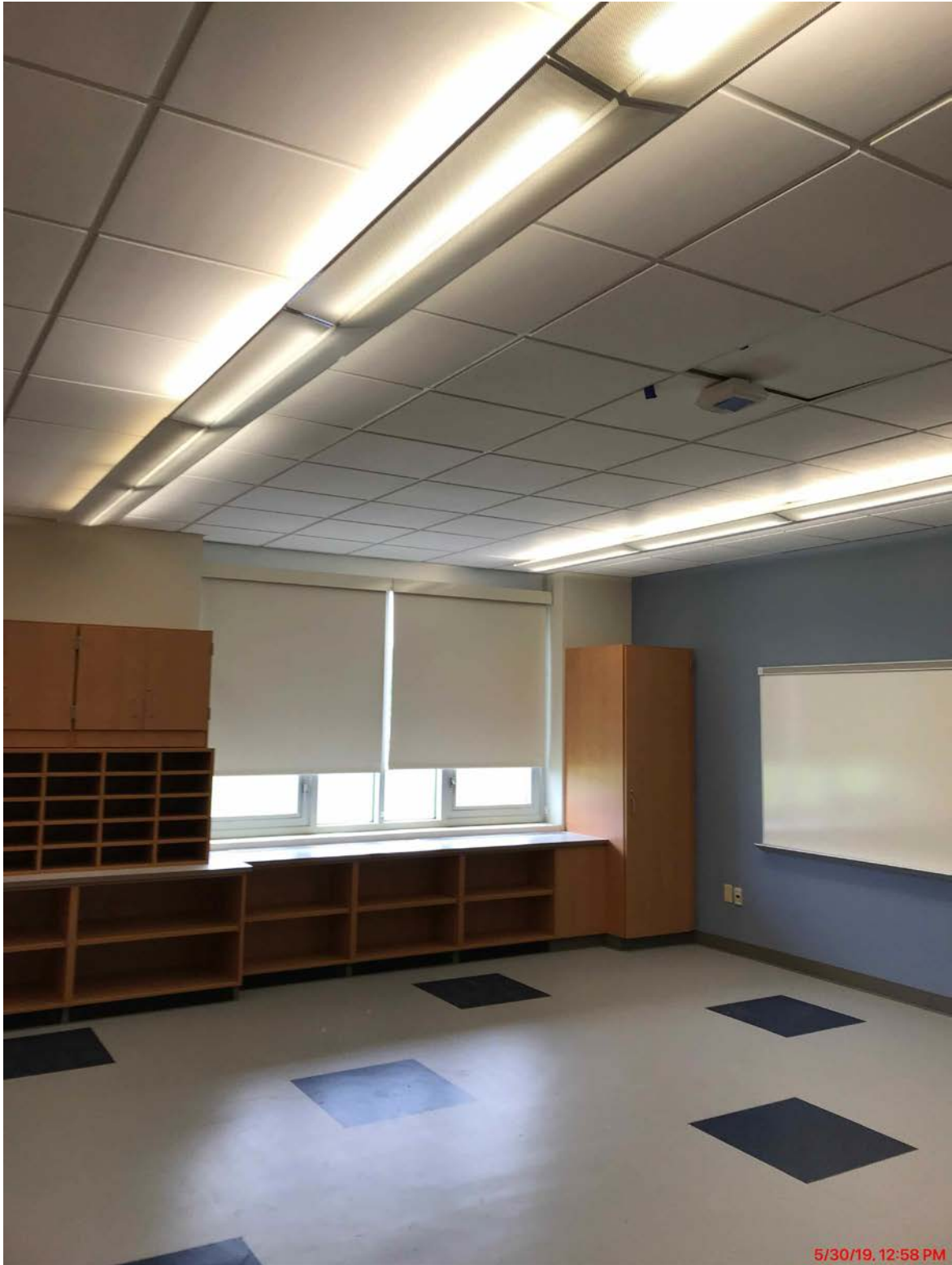
Eight New Elementary Classrooms Near Completion
