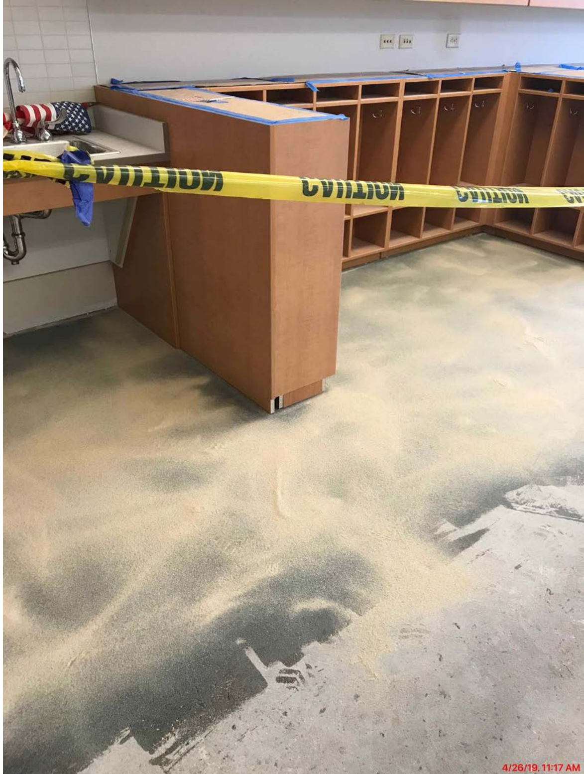
Glue Applied for Tile Installation in Eight Elementary Classrooms
