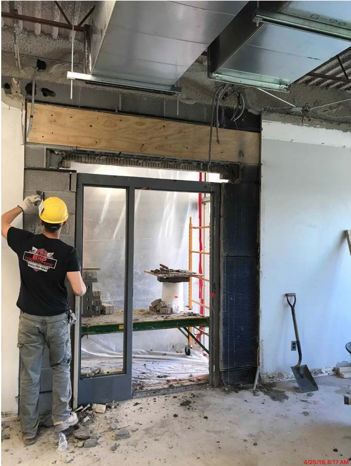
Installation of District Office Entry Door
