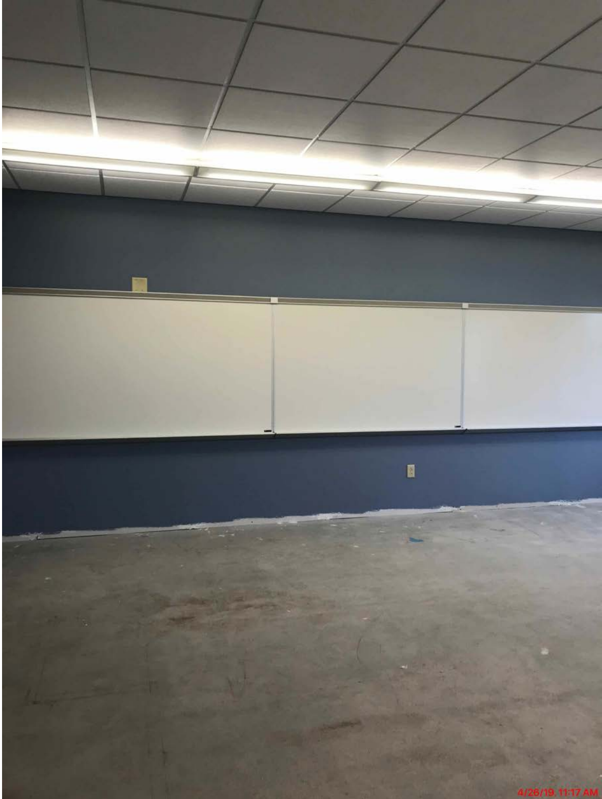
White Boards Installed in Eight Elementary Classrooms
