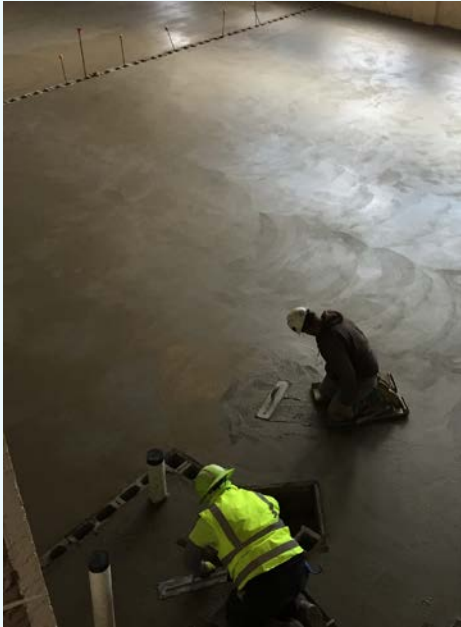
First floor slabs.
