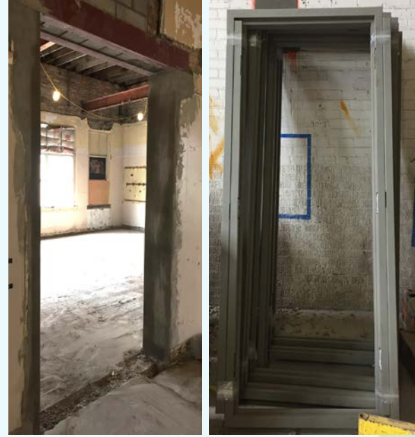
Door openings & frames ready.
