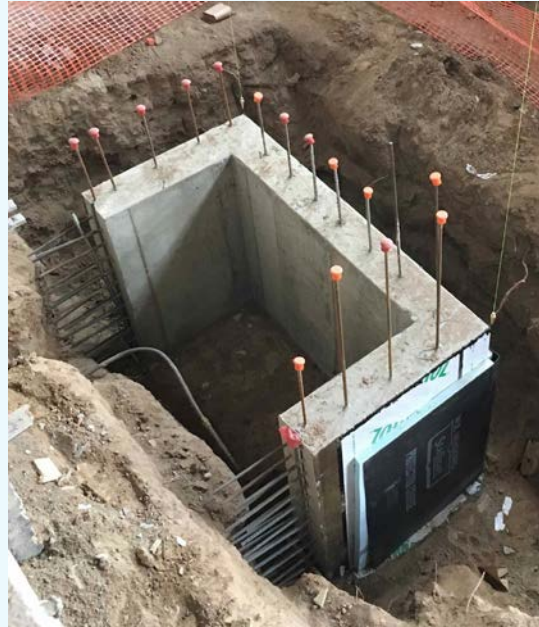
Pit for new elevator.
